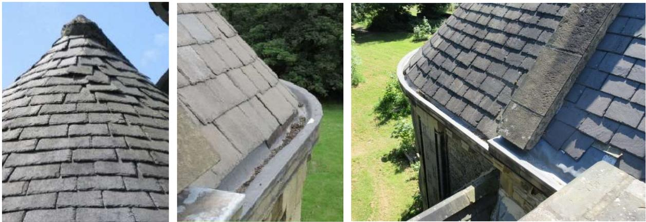
14. At abutment to the low stone Choir E wall cover flashings over soakers. Minor cracks in cement pointing of flashings, which tends to shrink. Lower flashings substitute after theft. Upper flashings remain old lead.
