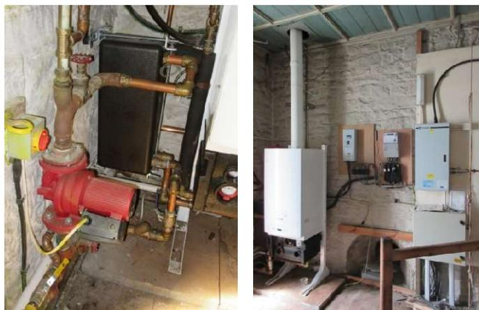
127. Two pipe circuit with variety of heat emitters. In Office timer, switch for fan convectors and frostat. Boiler thermostat, no room thermostat. Used Sundays only and said effective but expensive.
