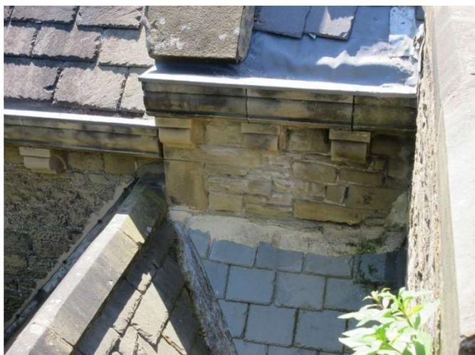
2023 – slate above Choir gutter, down pipe and Sacristy slate head flashing all missing
