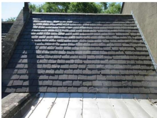
18. Between the **Sacristy** and the much higher later Organ chamber wall a box gutter drains the Sacristy and part of the Choir. It traps leaves and silt and is hard to reach past the Organ downpipe. This valley let water into the timbers below, causing current need for structural repairs (para 79). Previously lead, now substitute. Hard to see but the gutter appears complete and clean. The substitute flashing, previously loose from the Organ wall, now appears secure.
