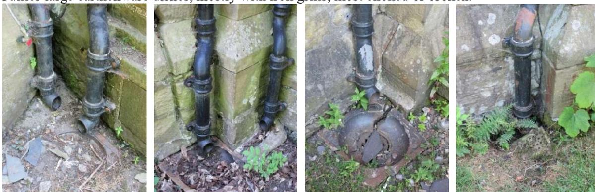
Most gullies are choked or broken, so rainwater more likely to soak into the ground and subwalls, adding to rising damp instead of running away safely to soakaways.
