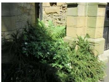
38. **N Vestry** plastic hopper and square pipe has been blocked (and damp damage on the stone and inside para 97). Check flow in rain and clear if needed. Gully blocked.
