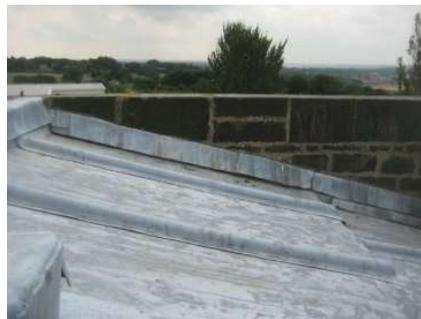
*The narrow top S bay had slipped about 1" down slope and was pushed part way back in 2013.*
