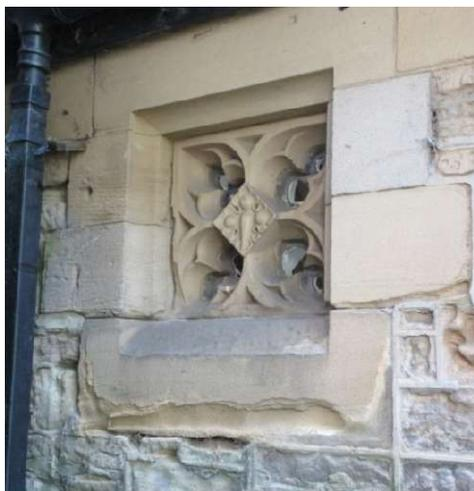
71. **Vestry** and **Office** tracery, mullions and sills obscured by clouded polycarbonate. Stone sound except minor damage at two Office mullions and Office W sill crudely repaired with mortar. Vestry door surround good but most ashlar joints open and some salts and surface decay at lintel (another sign of probable rainwater pipe blockage).
