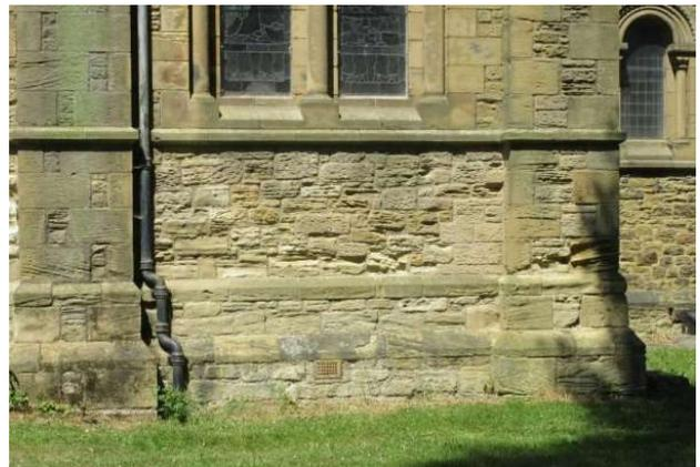
55. **Both Transept gables** have green streaks and minor open stone joints around and below the centre hoppers. Joints at the top of the buttresses below the hoppers are also open. May cause enough leakage to flake the paint inside (para 35).
