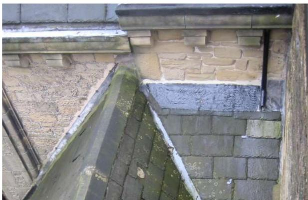
2008 – down pipe and (paint disguised) head flashing where Sacristy roof joins Choir
