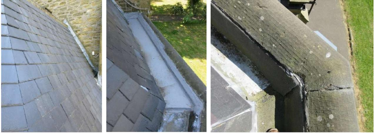
28. The N Vestry W side gutter has been painted over with sealant.
