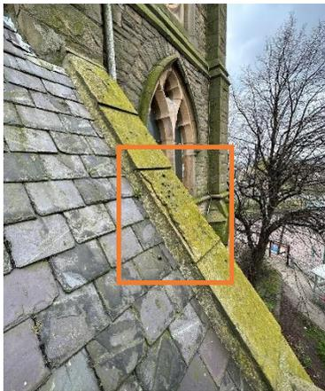
Figure 4- Coping stone delamination
