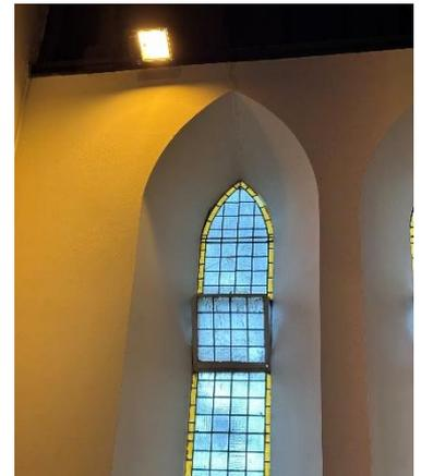
Figure 24 – window with hopper and cracked pane
