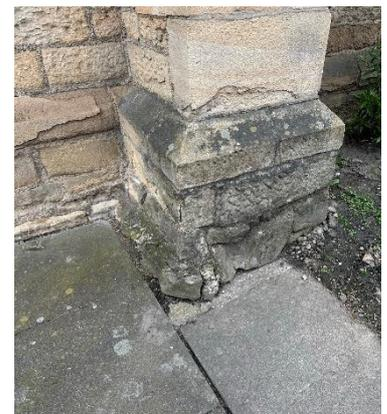
Figure 9 - erosion to base of buttress
