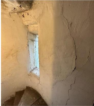
Figure 15 - crack to stair
