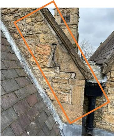
Figure 10 - crack to kneeler at 8.9
