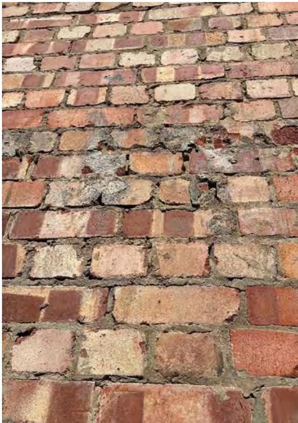
Example quality of brickwork
