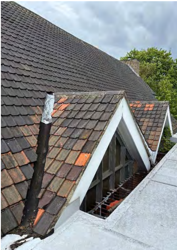
Lightwell Void Roof Area
