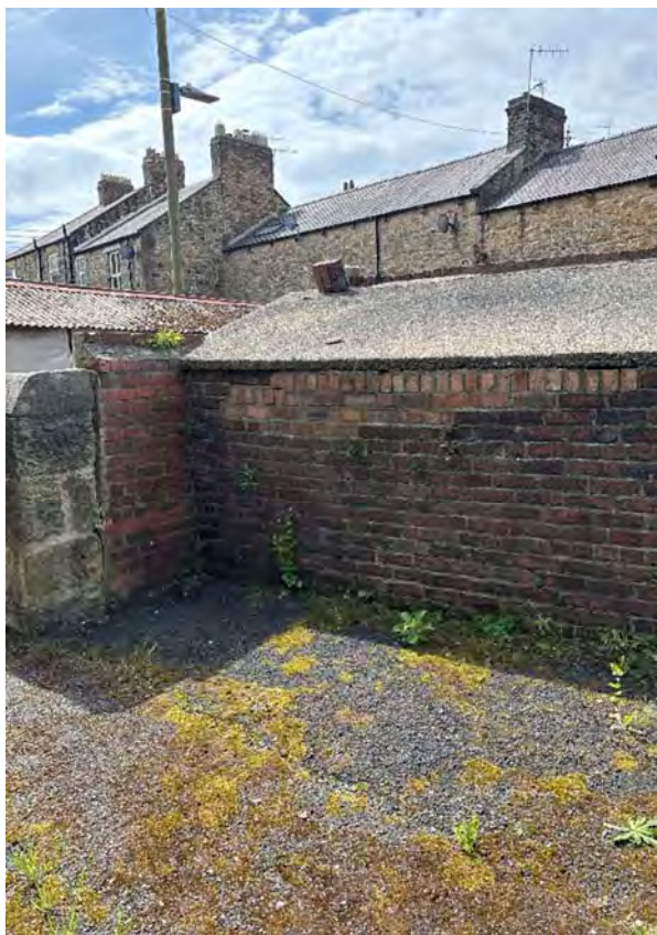
Overview of Brick Wall and Roof
