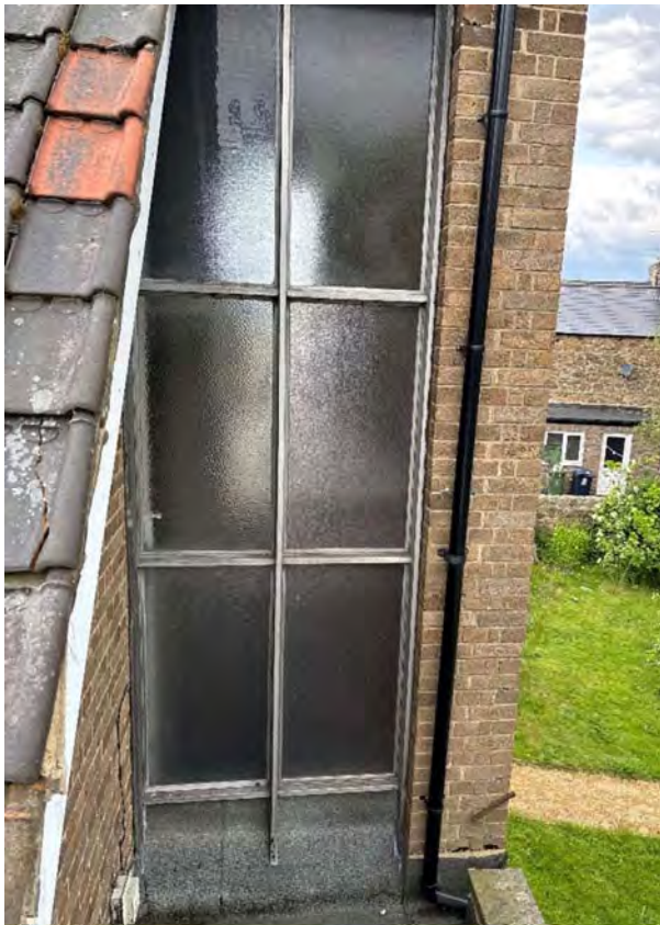
NW2 Overview (from Hall Roof)
