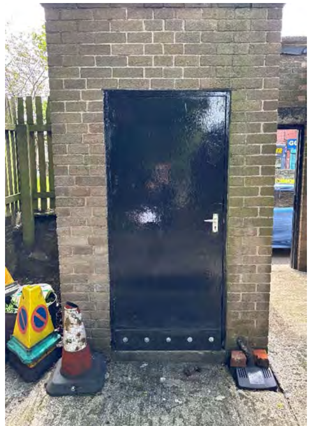
Overview of Door to External Store
