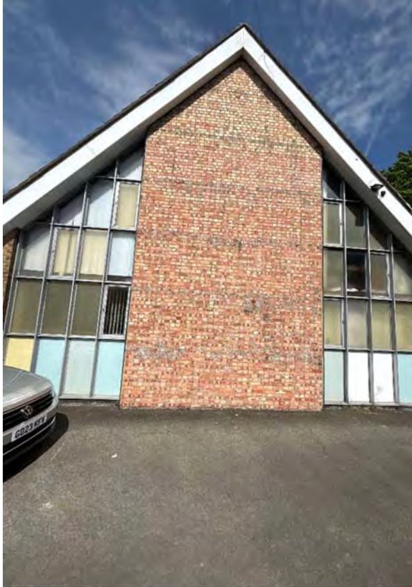
South Elevation overview
