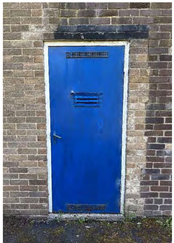
Overview of Boiler House Door
