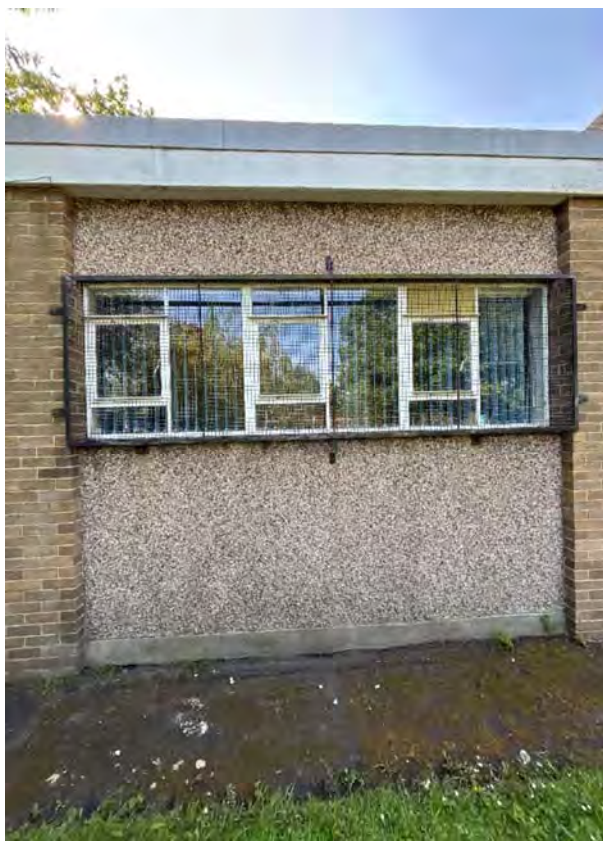
Overview of Hall North Elevation
