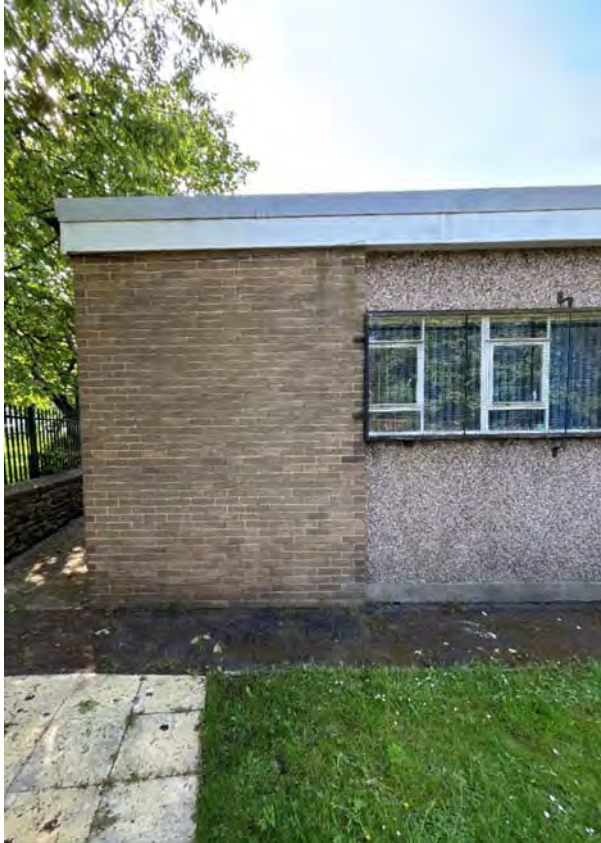
NW1 Overview (Left Side)
