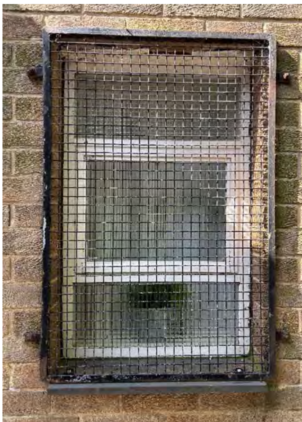
Overview of EW7 (Acc. WC Window)
