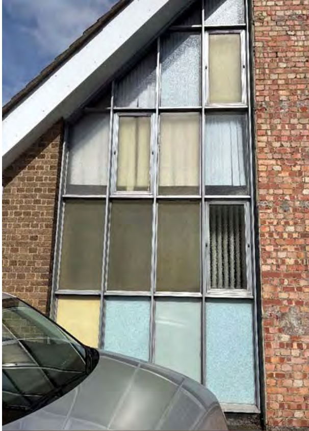
SW1 – Left Side Curtain Wall (South)
