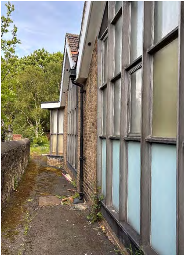
West Elevation Window Overview
