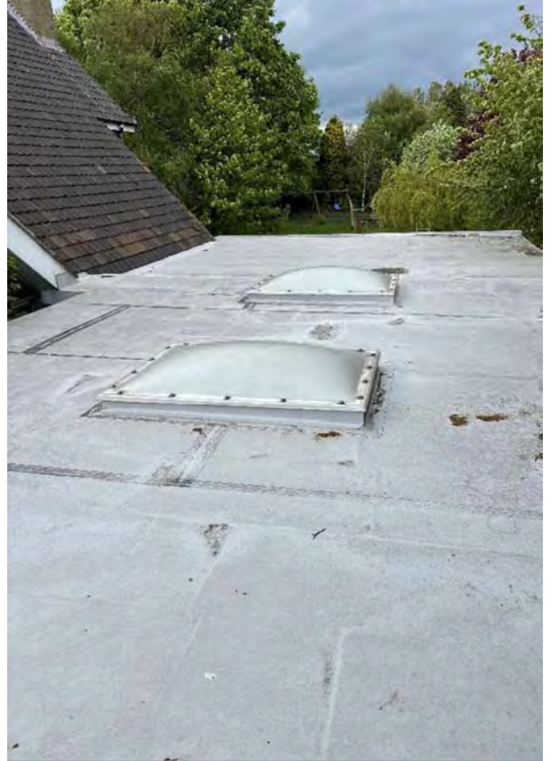
Overview of Hall Roof and Rooflights
