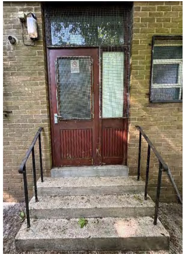
Overview of concrete steps.
