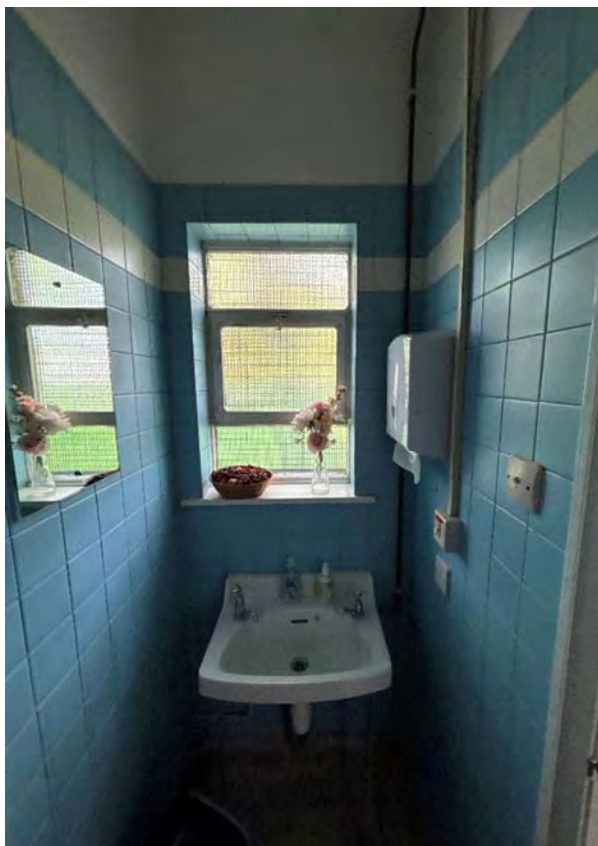
Overview of WC Sink Area.
