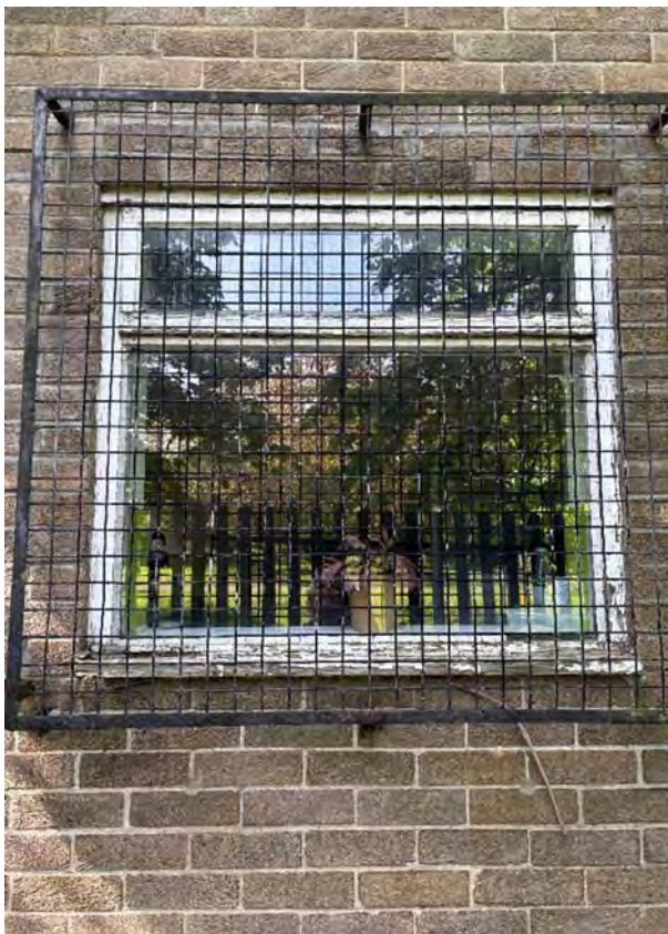
Overview of EW3 (Kitchen Window)
