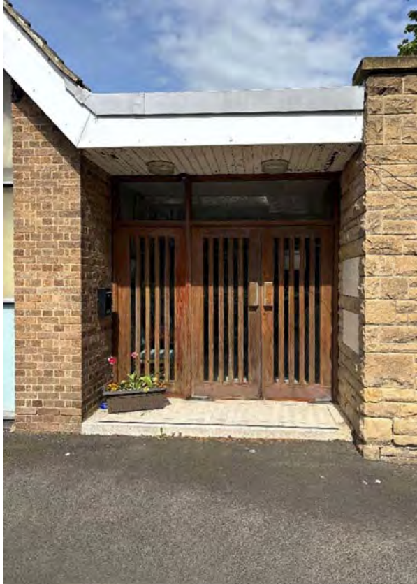
Overview of External Entrance Doors
