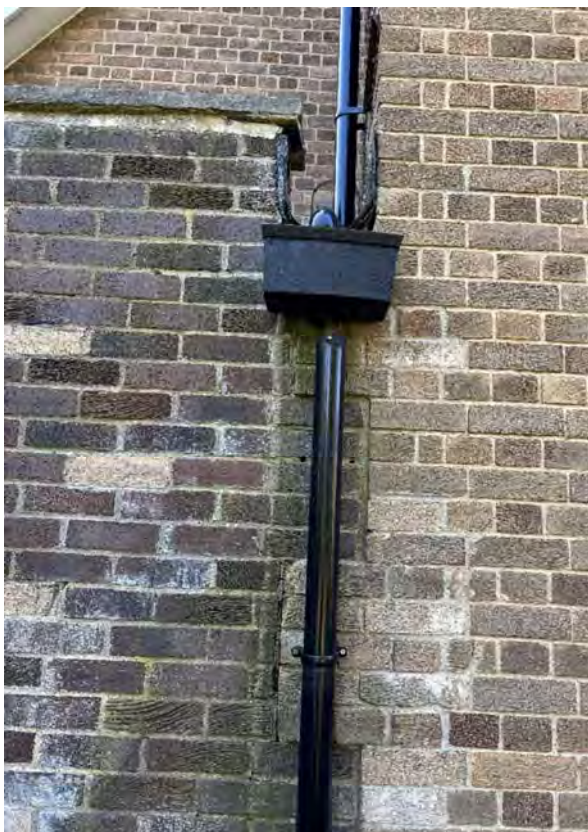
Downpipe to Boiler House Elevation discharges directly onto ground.
