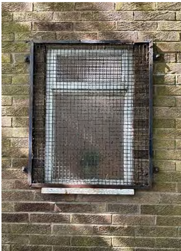
Overview of EW5 (Hall Window)
