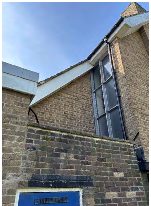
Area to top of boiler house elevation.
