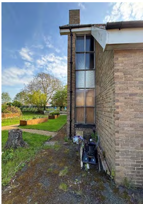
Overview of return north elevation for window.
