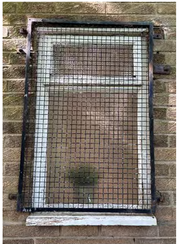
Overview of EW4 (Hall Window)
