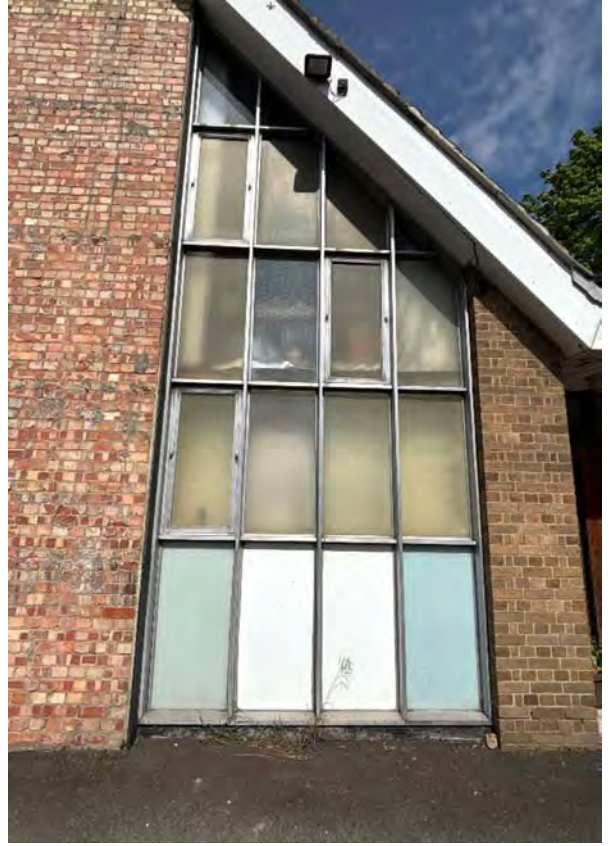
SW2 – Right Side Curtain Wall (South)
