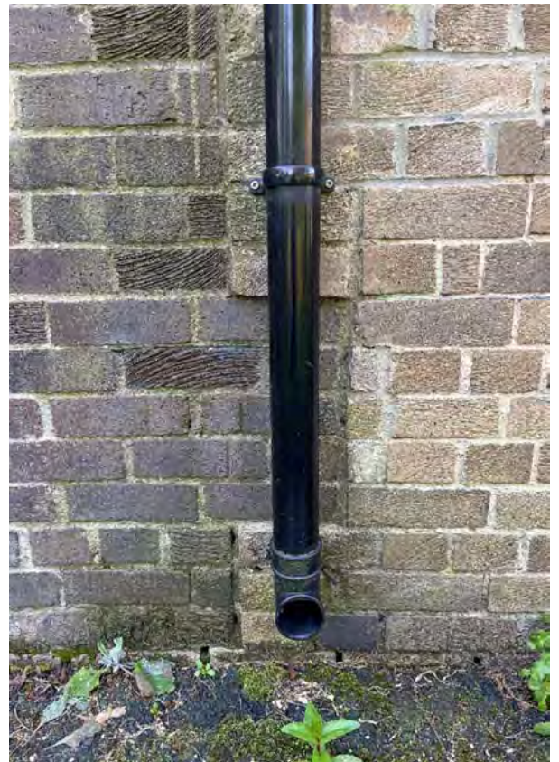
North Elevation terminates onto ground.
