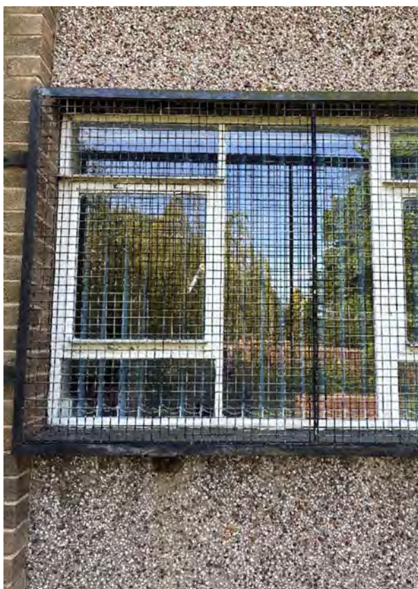
Metal covering to window
