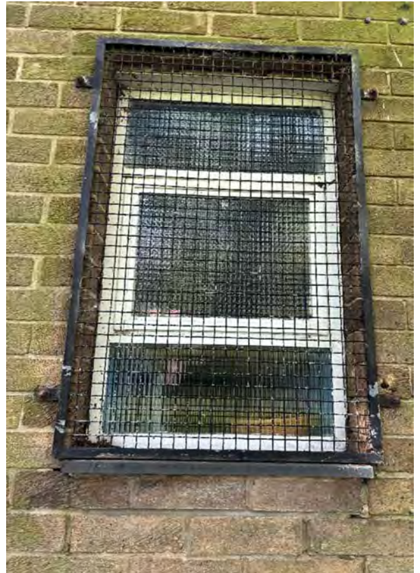
Overview of EW2 (WC Sink Area)
