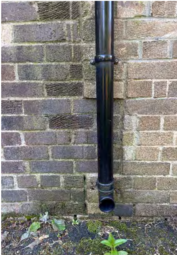
Downpipe to Boiler House Elevation discharges directly onto ground.
