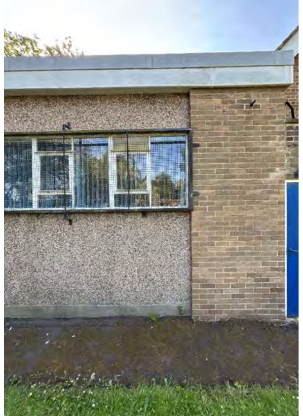
NW1 Overview (Right Side)
