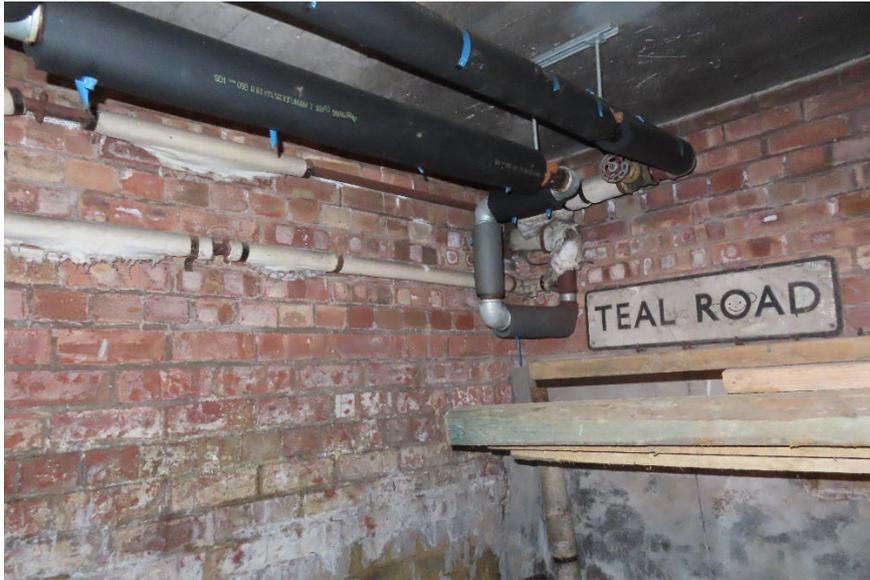
*Photo 23, Disturbed old insulation to boiler room, possibly asbestos*
