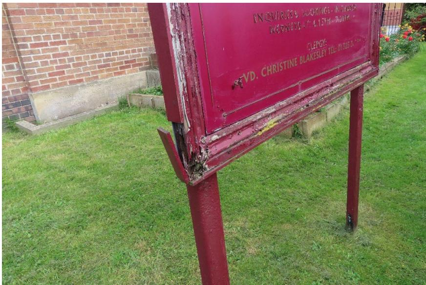
*Photo 32, decaying timber and poor decoration of sign board*
