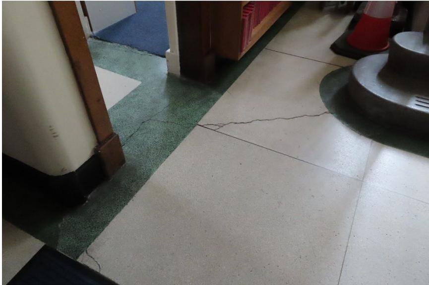
*Photo 27, Crack to entrance floor*
