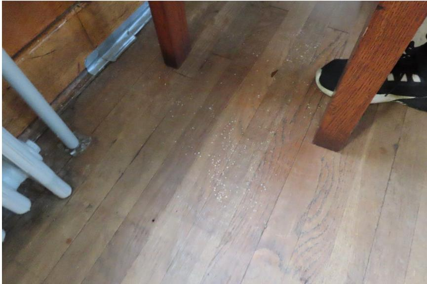
*Photo 29, Evidence of infestation of floor boards*
