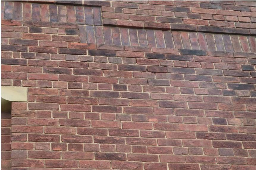
*Photo 15, Example of area of erosion to pointing*
