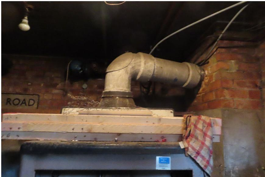
*Photo 24, cement flue to old boiler possibly asbestos*
