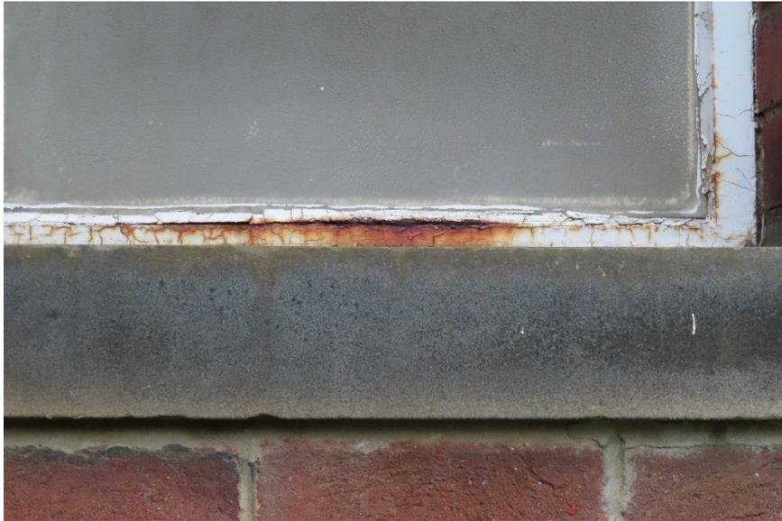
*Photo 19, Corrosion and poor decoration to steel Crittal window*
