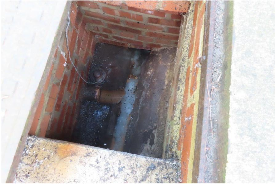
*Photo 33, Blocked drain adjacent to entrance gate*
