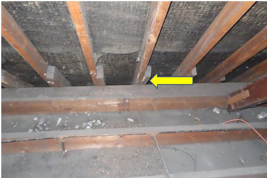
*Photo 30, evidence of infestation of rafters above purlin*
