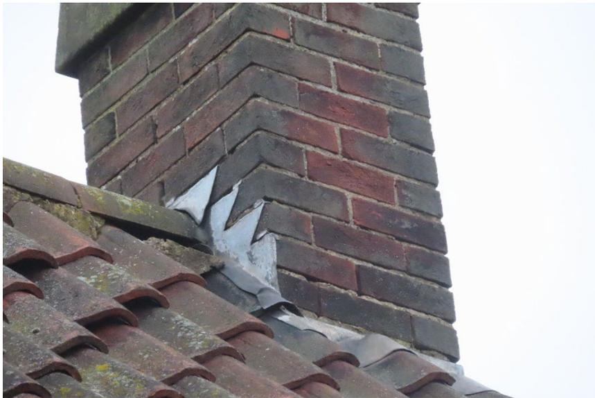
*Photo 10, condition of chimney stack pointing*
