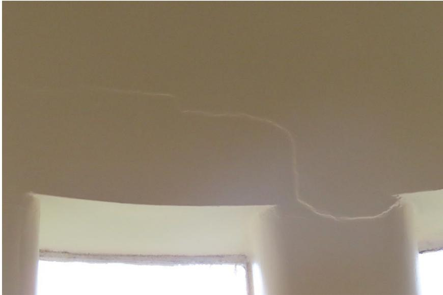
*Photo 25, repaired crack over stairwell window*
