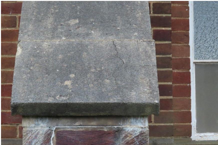
*Photo 12, crack to capping stone of buttress 2*
