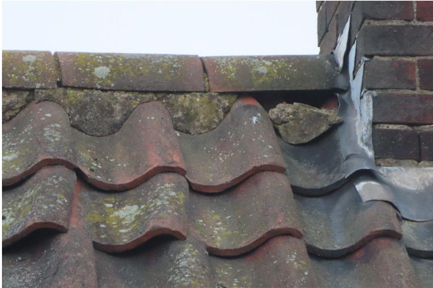
*Photo 9, Example of loose mortar bedding to ridge tiles*
