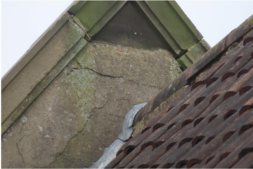
*Photo 13, Cracking to render on inside face of South gable*
