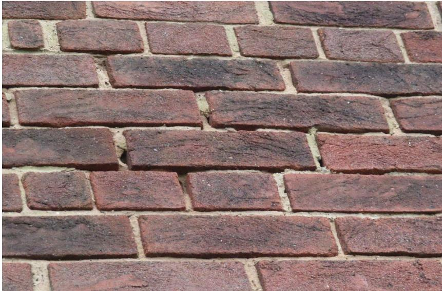
*Photo 16, Example of area of erosion of pointing*
