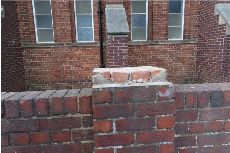
*Photo 31, Example of damage to boundary walls*
