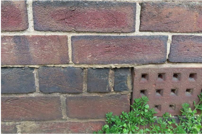
*Photo 17, oversailing of brickwork at DPC level between buttresses 7 & 8*
