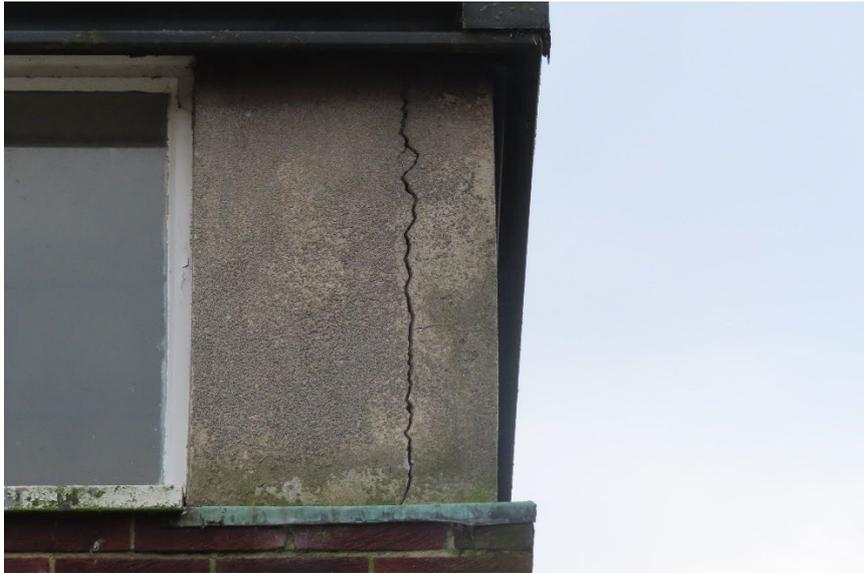
*Photo 21, example of crack to render over structural frame of the Hall at high level.*
