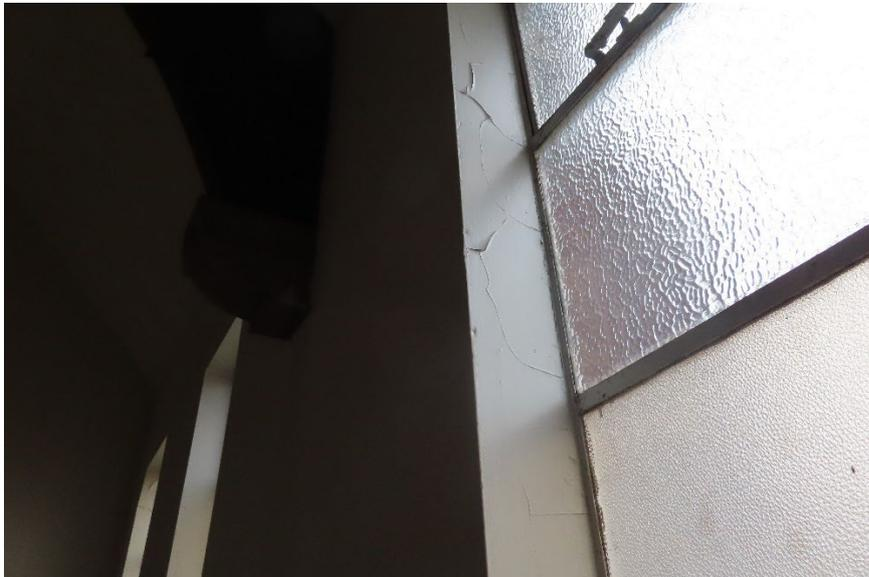
*Photo 22, example of cracking to internal paint finish*
