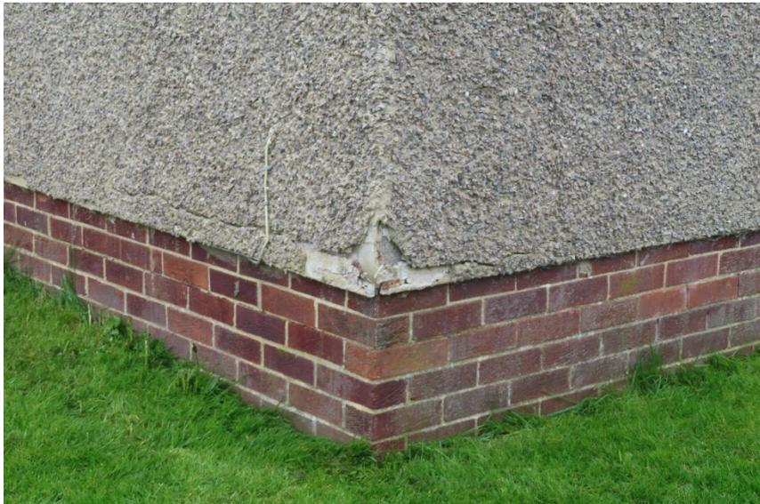
*Photo 18, Cracked and delaminated render*
