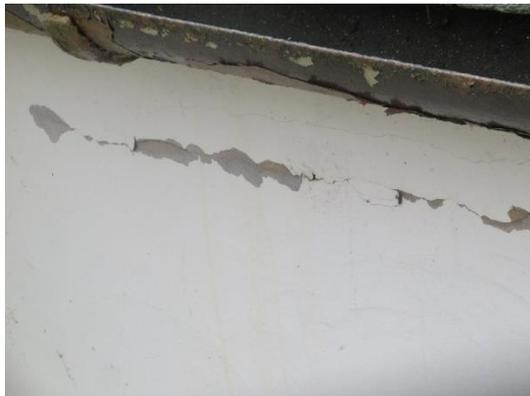
*Photo 18, Example of horizontal cracking under rainwater gutters*
