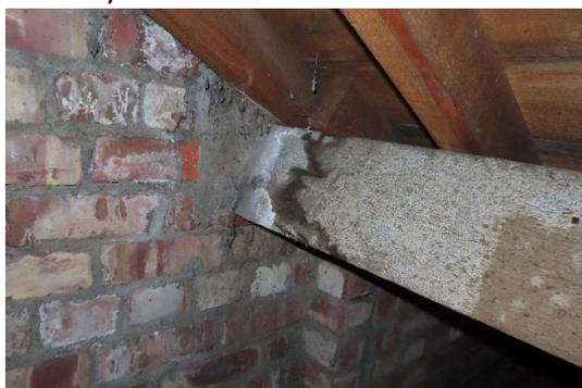
*Photo 28, Evidence of water staining to purlin ends*
