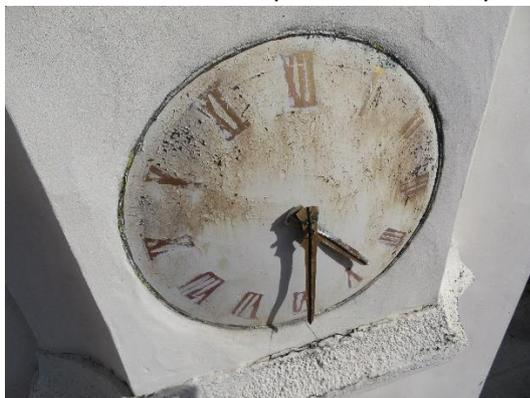
*Photo 23, Deterioration of finish to clock face*
