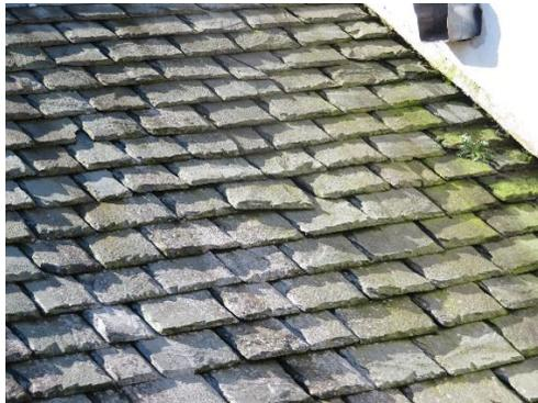
*Photo 2, Example of slipped slate to north elevation*
