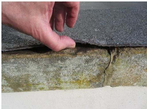
*Photo 6, Lifting felt to Vestry parapet*
