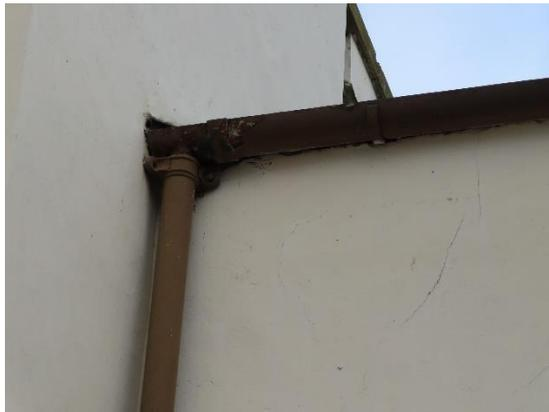
*Photo 10, Displaced gutter joint*
