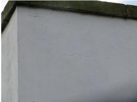
*Photo 12, Crazed cracking to render*
