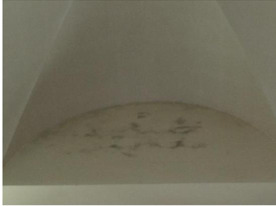
*Photo 33, Mould to arched sections between frames*
