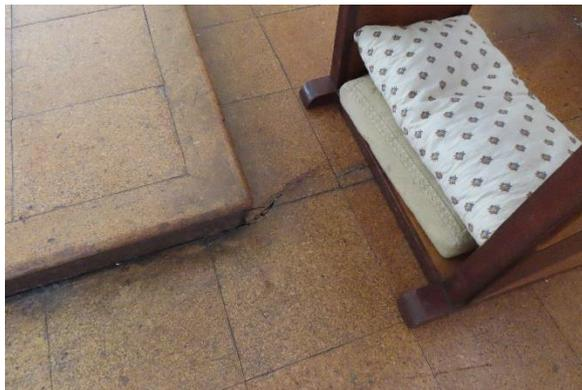
*Photo 36, Cracking to cork tile at corner of altar*
