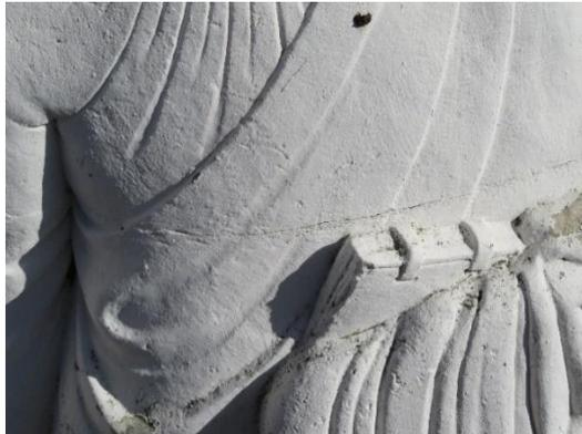
*Photo 22, Cracks at the junction of the statue elements*
