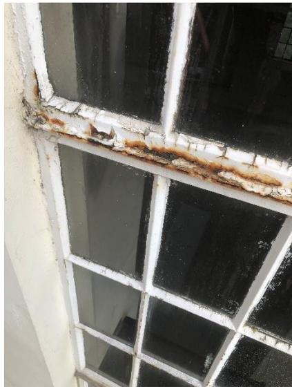
*Photo 25, Example of corrosion to window frames*
