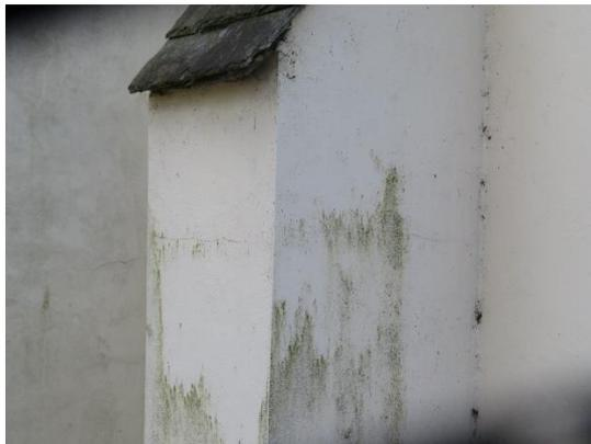
*Photo 17, Regular spaced cracking to render on buttresses visible externally and internally*
