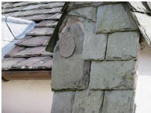
*Photo 4, Example of slipped slate to buttress*
