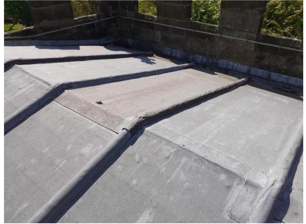
*Tower Roof: Lapped ridge with patch repairs*
