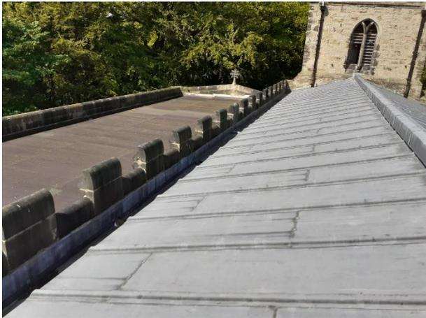
*Nave roof south pitch in lead rolls with ventilated ridge and south aisle in stepped bitumen felt*
