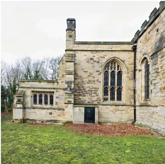
*East Elevation: severe stone erosion.
