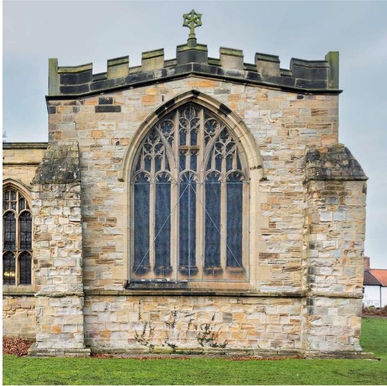
*Chancel East Elevation: severe stone erosion.
