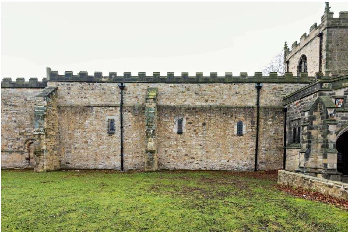
*North Elevation of Nave: oldest masonry below the string line.*
