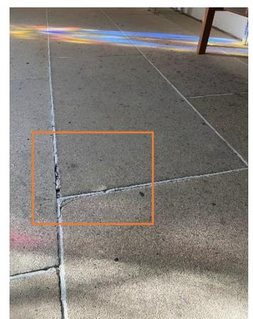
Figure 22 – Floor lifting
