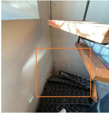
Figure 17 – SW Corner with damp and hairline cracks
