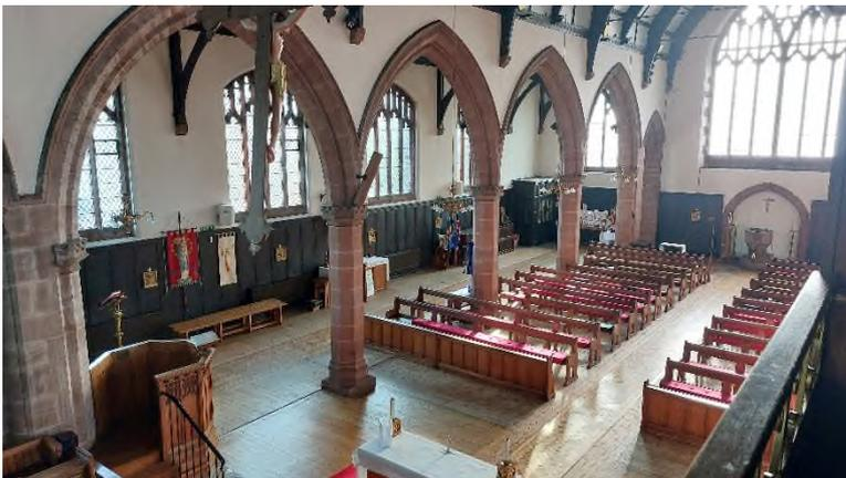
The arcades are lancet arched in exposed masonry and there is no evidence of cracking or movement to them. The arches are supported by octagonal stone columns that features castellated capitals and moulded bases and there doesn't appear to be any damp rising up from them.
