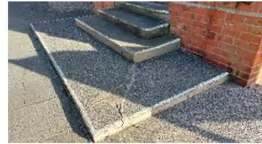
The north boundary is where the parish hall is. The area between the two buildings is paved again, slightly sloping towards the church hall with a gravel margin up against the north aisle. The stone steps leading up to the north door are sloping downwards slightly and the middle stone step is loose, and the bottom concrete margin is cracked causing a trip hazard.
