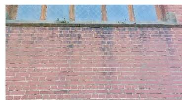
At the east gable of the Lady Chapel, the dampness in the wall around the window opening would appear to be because of defective pointing of the brickwork adjacent to the top of the south buttress, rather than a roofing problem.
