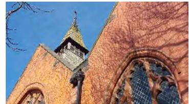
Timber framed fleche with square spire of Westmoreland slating with button capped lead finial top with rusty cross above and the lighting conductor comes down from the cross down on the western side. Hip slate missing at NW side and there are slates fallen into the parapet gutter, reports Ferguson.
