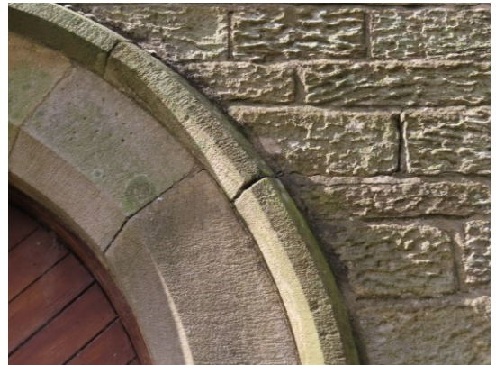
Failing finish to East Vicars Vestry door (left) and open joints and cracking above the door (right)
