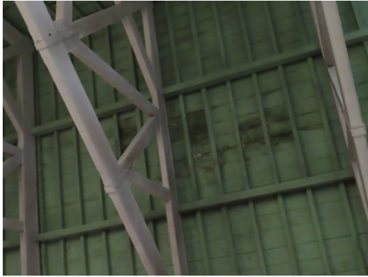
Damp staining to sarking boards of the Nave including near the bell rope (right)
