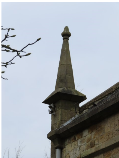
Open/hungry joints to West pinnacle on the south side of the Nave
