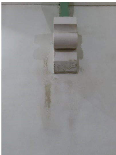
Mildew growth to the North Nave wall above and below left
