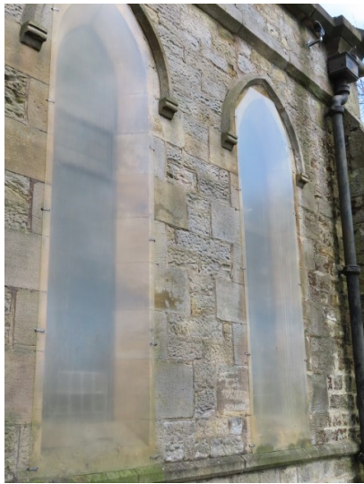
Aging protection is becoming discoloured with some algal growth further obscuring the protection
