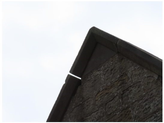
Open joints to the water table on the organ chamber
