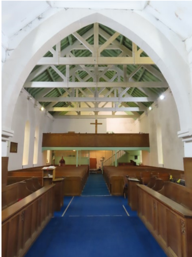
General View of the Nave from the Chancel
