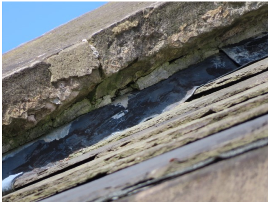
Failing mortar to chase over flashings to South West of the Nave (left) and bellcote (right)
