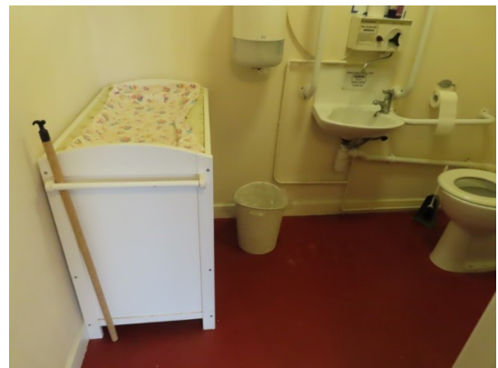
Bulky changing table taking up to floorspace in the Accessible WC
