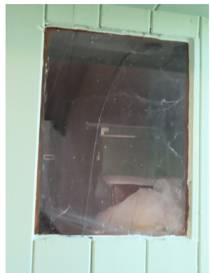
Cracked pane to understairs cupboard
