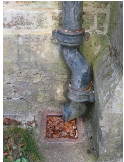
Rusting downpipes, vegetation growth, leaf build up (above and below left) and to the top left, downpipe not fully discharging over gully
