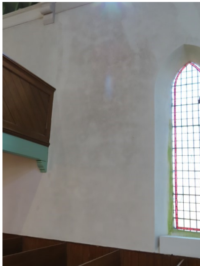
Mildew growth to the North Nave wall above and below left
