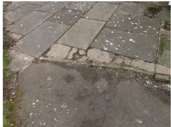
Open joints to paving up to Parish room and the concrete to the edge of the ramp (non-compliant) is breaking up
