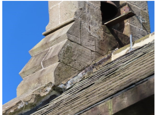
Failing mortar to chase over flashings to South West of the Nave (left) and bellcote (right)
