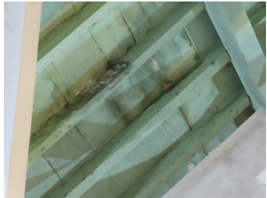
Damp staining to sarking boards of the Nave including near the bell rope (right)
