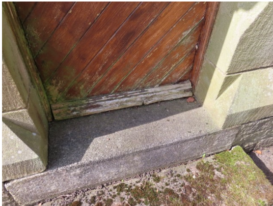
Failing finish to East Vicars Vestry door (left) and open joints and cracking above the door (right)
