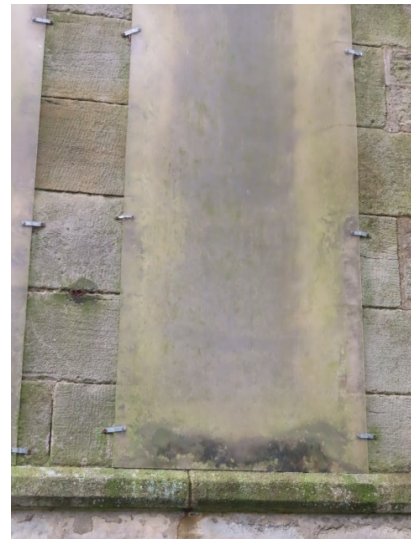
Aging protection is becoming discoloured with some algal growth further obscuring the protection
