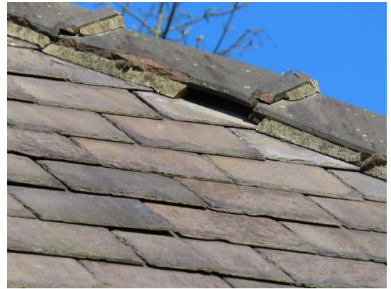
Failing and missing mortar bedding to the hops of the parish room
