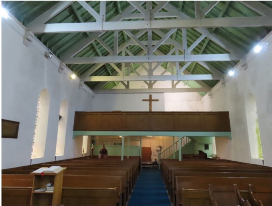
General View of the Nave and gallery looking West
