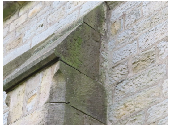
Failing mortar and open joints to the North Nave and buttress
