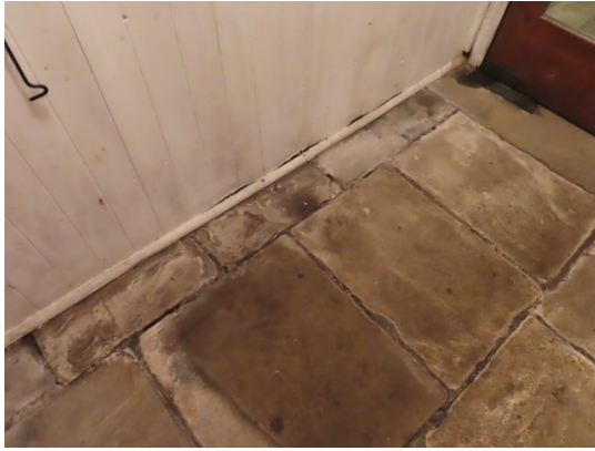
Lower edge of the porch boarding is warped lining of the porch
