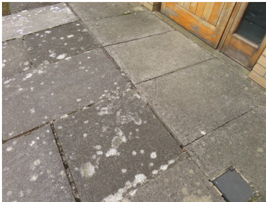
Open joints to paving up to Parish room and the concrete to the edge of the ramp (non-compliant) is breaking up
