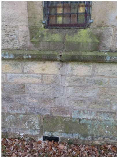
Open joints and cracking to sill of window Nv (left) and cracking and weathered stone over the same window (right)
