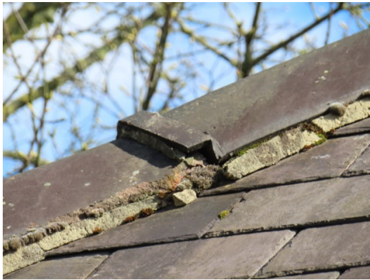
Failing and missing mortar bedding to the hops of the parish room
