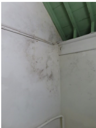
Dampness and blistering to plaster near the gallery stairs
