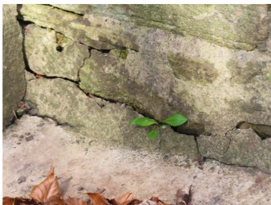
Cracking and vegetation growth to South Nave (left) and South Chancel (right)
