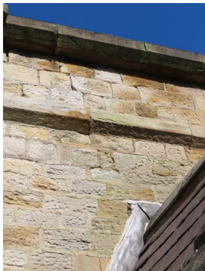
Cracking and open joints to South Nave
