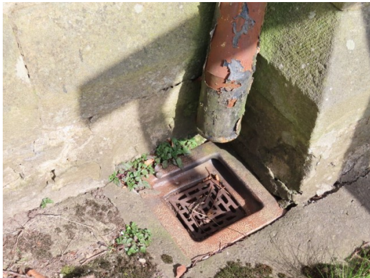
Rusting downpipes, vegetation growth, leaf build up (above and below left) and to the top left, downpipe not fully discharging over gully
