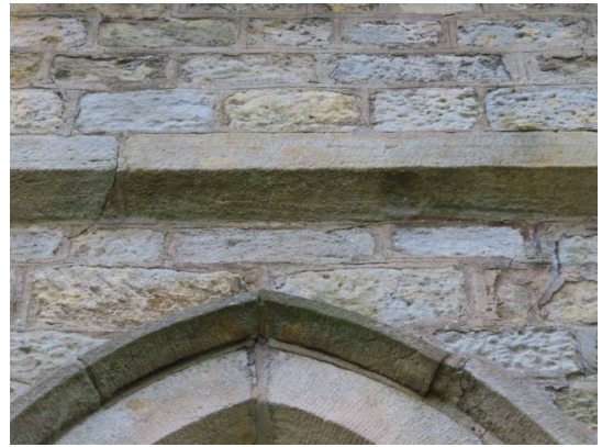
Open joints and cracking to sill of window Nv (left) and cracking and weathered stone over the same window (right)
