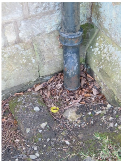
Rusting downpipes, vegetation growth, leaf build up (above and below left) and to the top left, downpipe not fully discharging over gully
