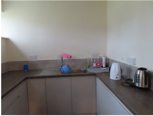
Sockets in the kitchen are very close to the sink/water source
