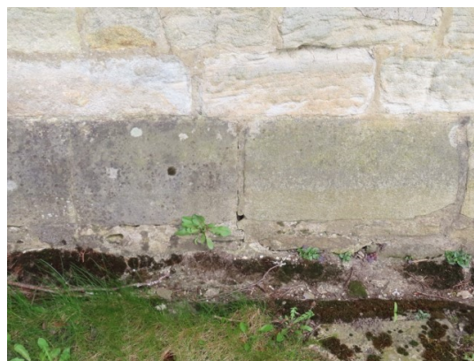
Cracking and vegetation growth to South Nave (left) and South Chancel (right)
