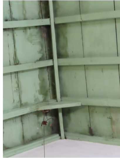
Damp staining to sarking boards of the Nave including near the bell rope (right)
