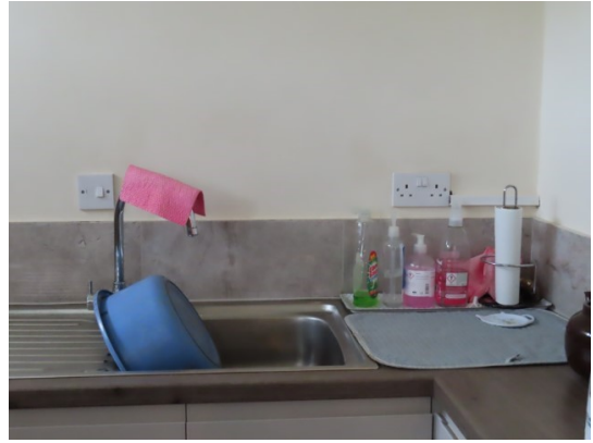
Sockets in the kitchen are very close to the sink/water source
