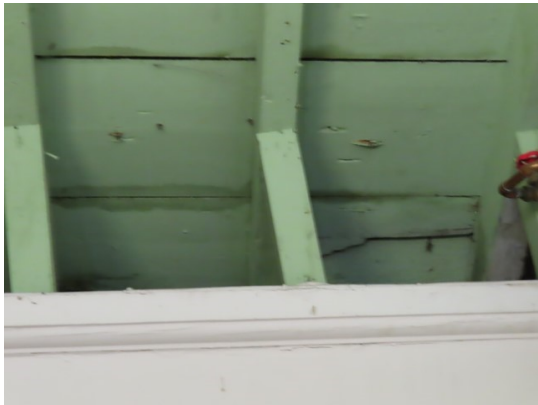
Damp staining to sarking boards of the Nave including near the bell rope (right)
