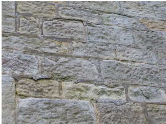
Failing mortar and open joints to the North Nave and buttress
