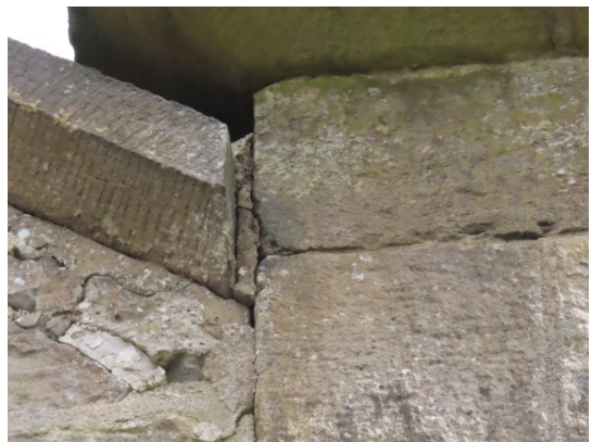
Open/hungry joints to West pinnacle on the south side of the Nave
