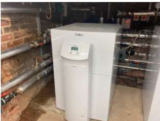
Internal heat pump unit that draws heat from ground
