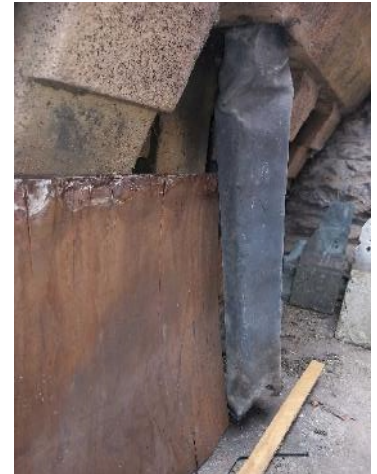
Damaged downpipe
