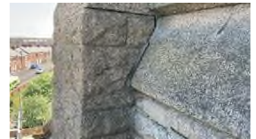
Open joints due to minor movement
