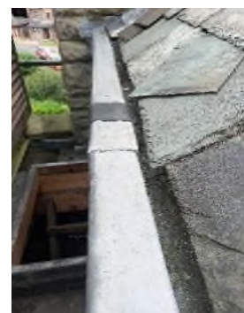
Damaged gutter
