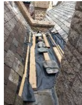
Missing lead gutter
