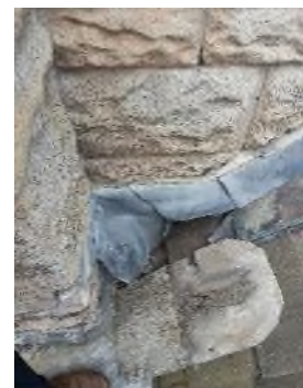
Missing flashings
