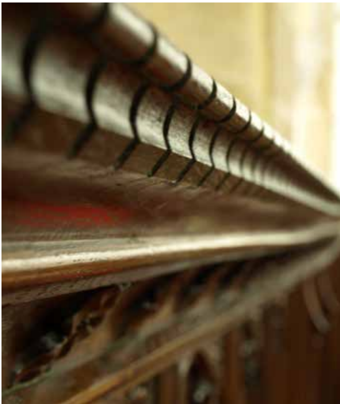
High quality joinery is a feature of the church, all generally in good condition
