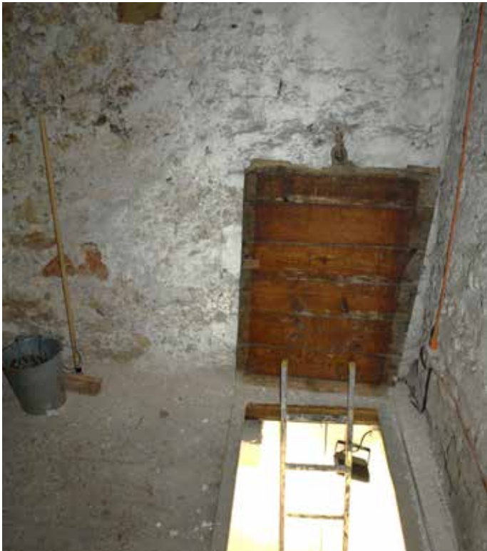
Peeling of impervious paintwork in tower - north wall, assumed drying out. Cement render internally in stage above requires removal
