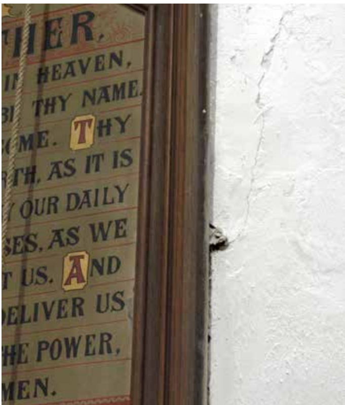
Loose fixings to Lords' Prayer board
