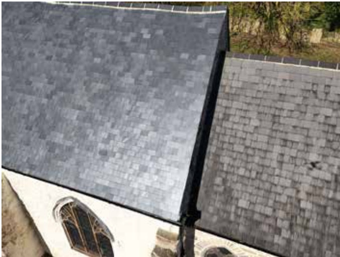
South roof slopes: contrast between new Spanish slate on nave (left) and Welsh slate on chancel (right)
