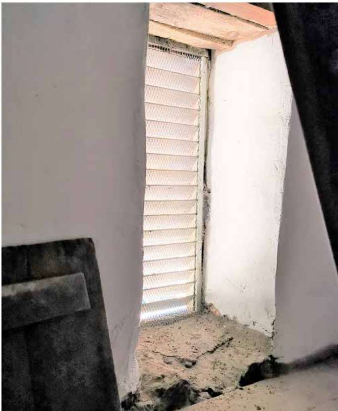
Lintels to south louvre still timber, in good condition. All others concrete. Metal grills in good condition, fixed securely
