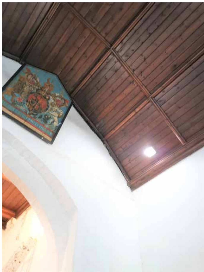
Nave ceiling boarded. Gap between ceiling and tower wall would benefit from clearing of debris and filling
