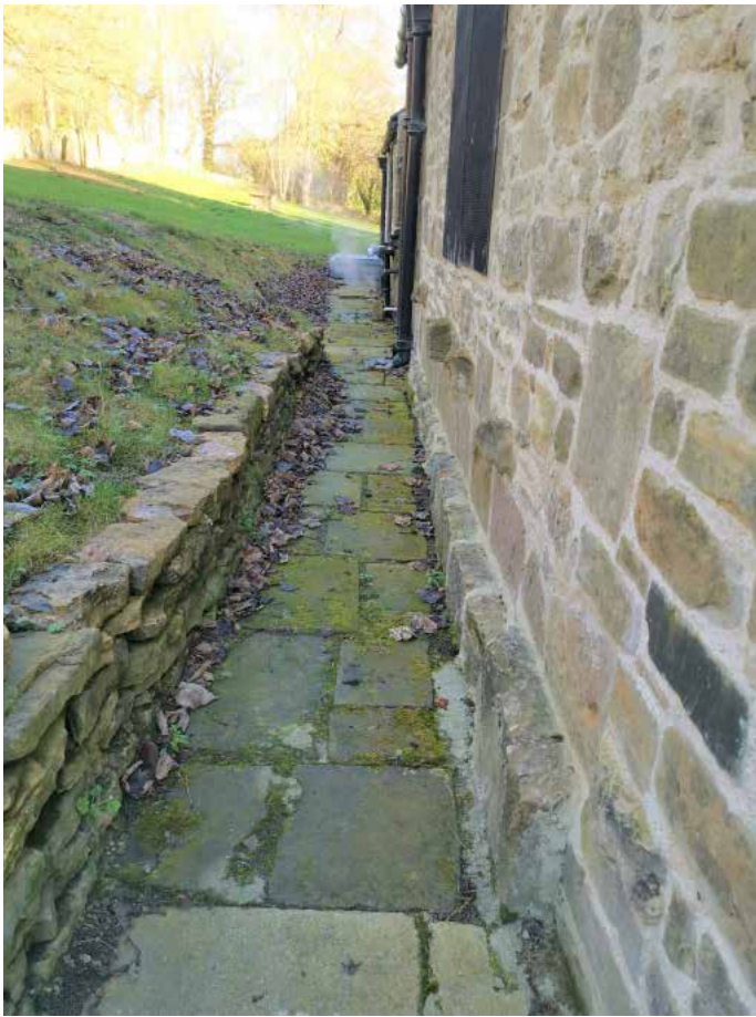
Hardstanding against base of wall will be trapping moisture - consider removal and laying grass directly up to base of walls
