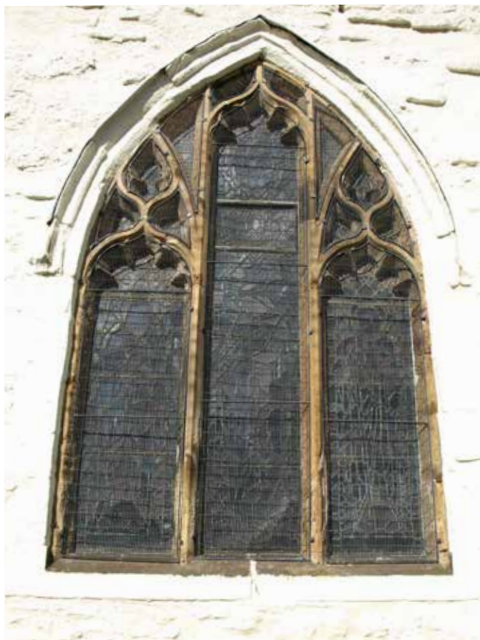
Window on south nave - stonework surrounds heavily deteriorated. Hoodmoulds now protected with lead
