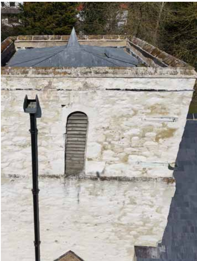
Wear and weathering of limewash finish
