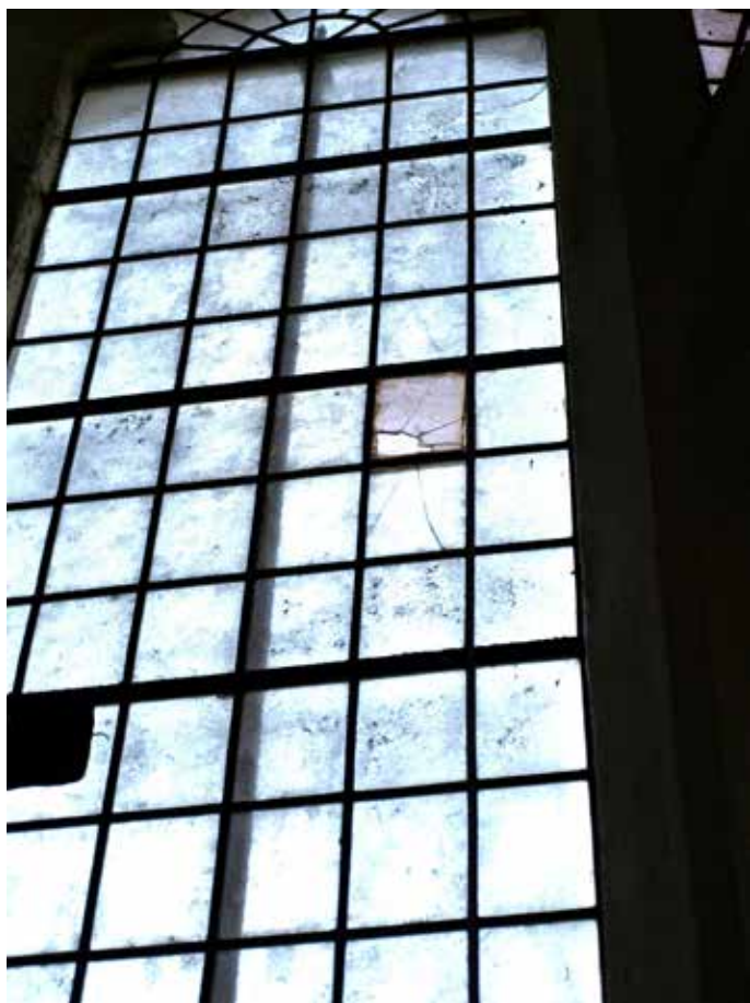
Window in north of nave has several broken square quarries and some leadwork distorted
