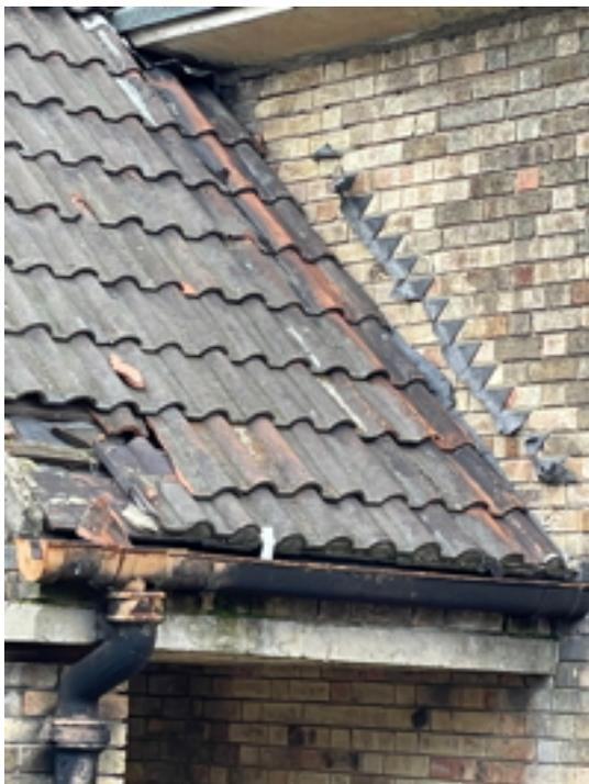
**Typical cast iron gutter and rainwater pipe to pantiled roof**
