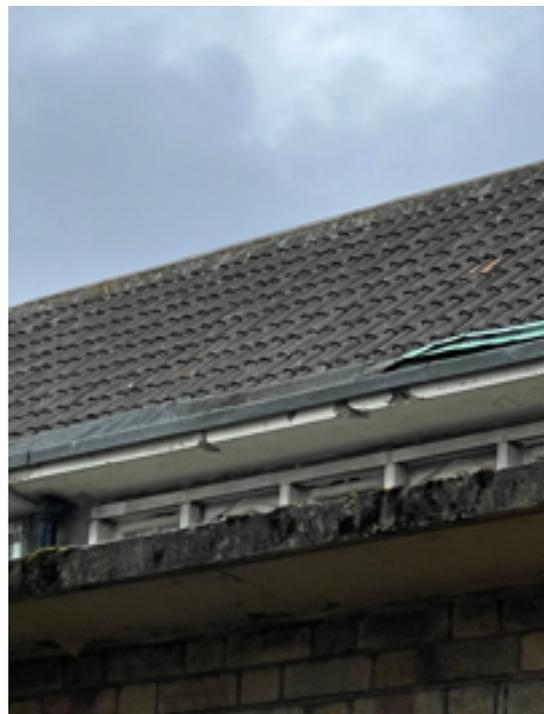
Spalling to concrete eaves
