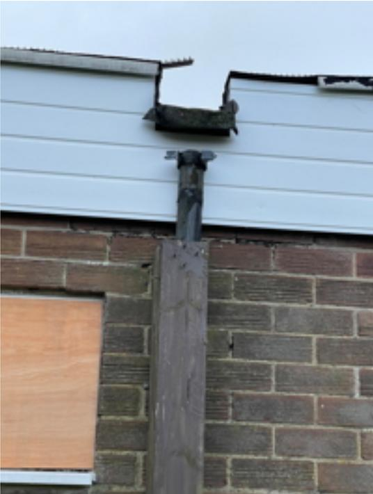
**Missing hopper head to Hall west elevation**
