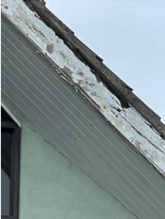
**Rotten verge boards east elevation**
