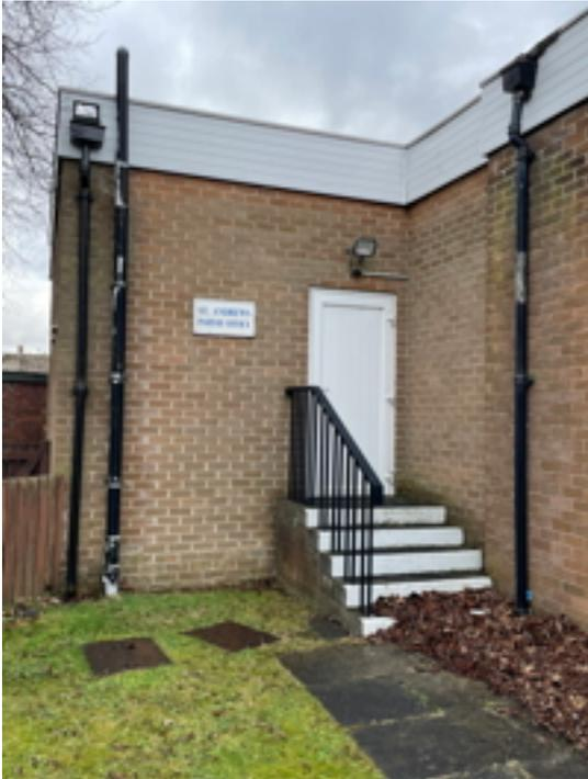
**Typical Hall rainwater pipes and hopper heads**
