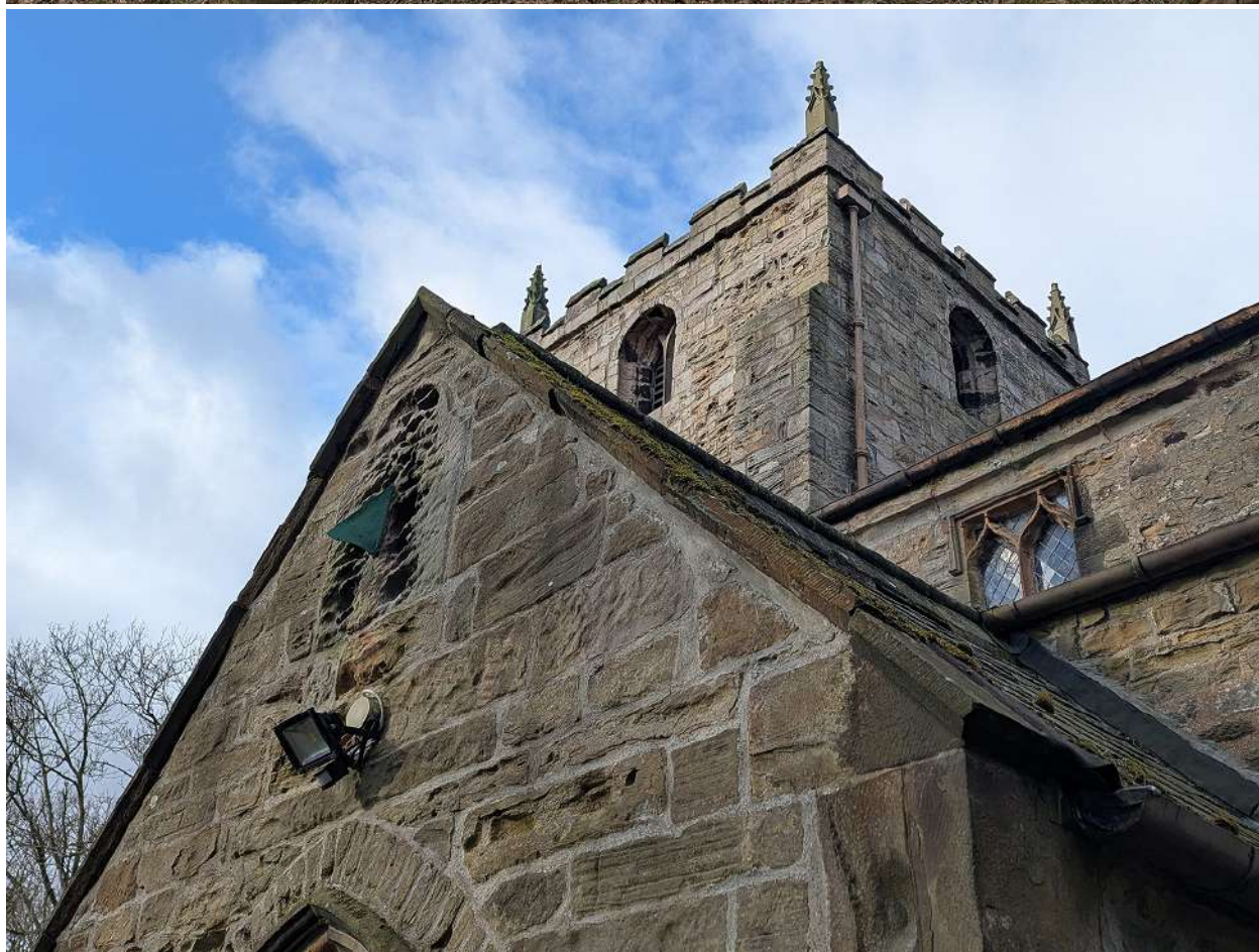
Fig. 4 | Church Photographs (4.1 - 4.4 Exterior)
