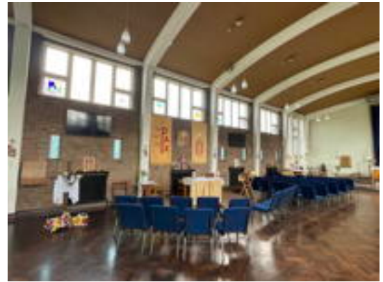
North Elevation Brickwork
