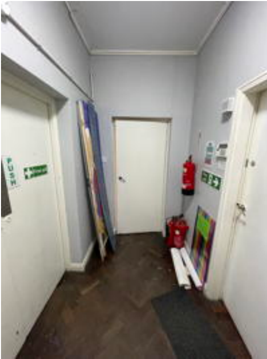
Vicar's Vestry South Lobby Looking North
