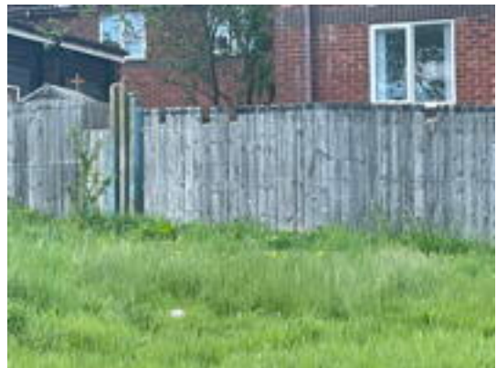
South Boundary Fence Towards Western Corner
