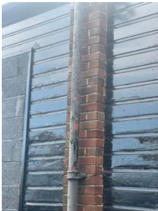
Hall Rainwater Pipe
