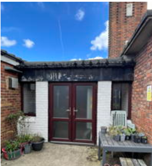
Link Lobby Doors
