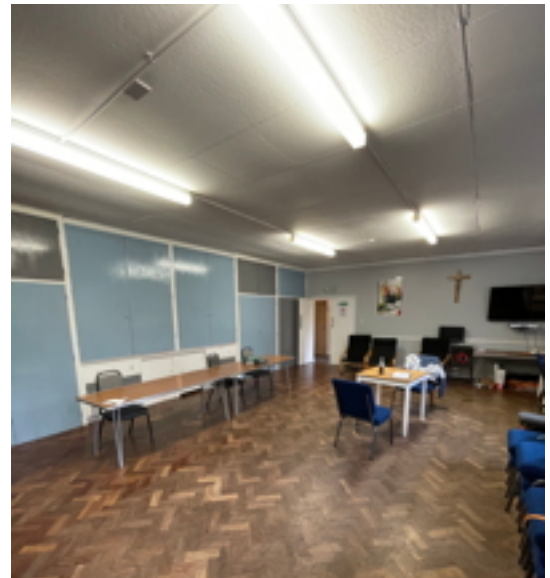
Fluorescent Type Lighting
