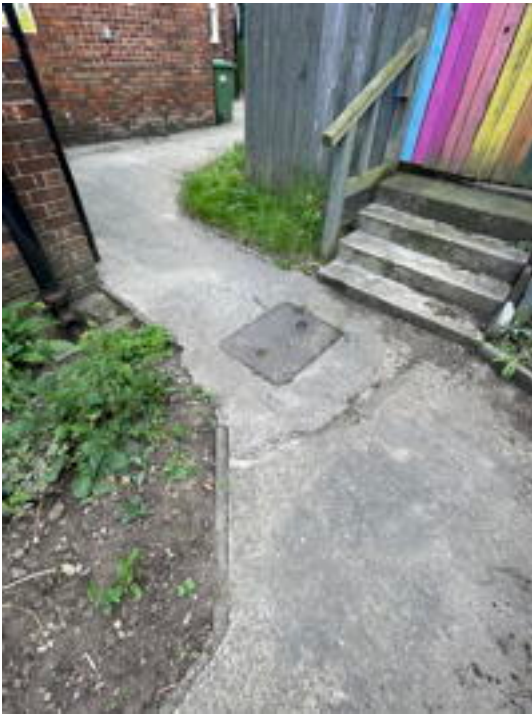
South Elevation Inspection Chamber
