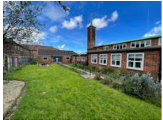
Enclosed Raised Garden to The South
