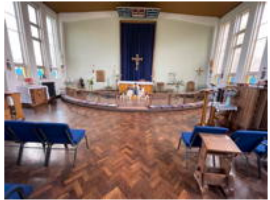
East End Wood Block and Stone Flooring
