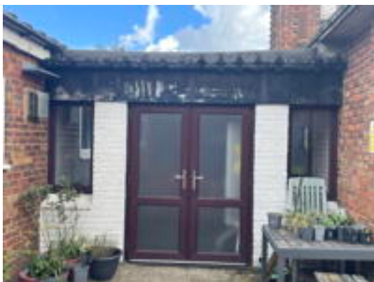
Felt to Link Lobby Roof
