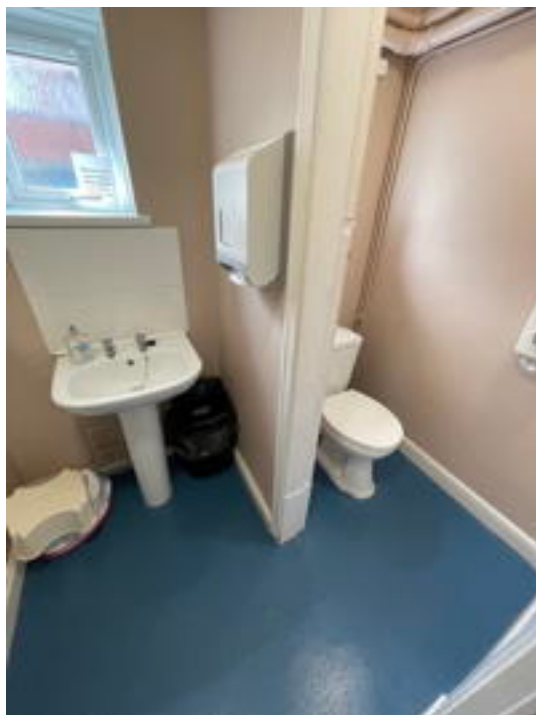
WC Looking South
