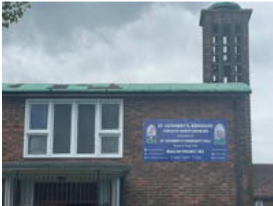
Patching to North Elevation Roof
