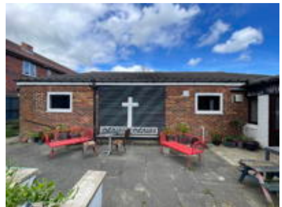
Hall East Elevation Windows
