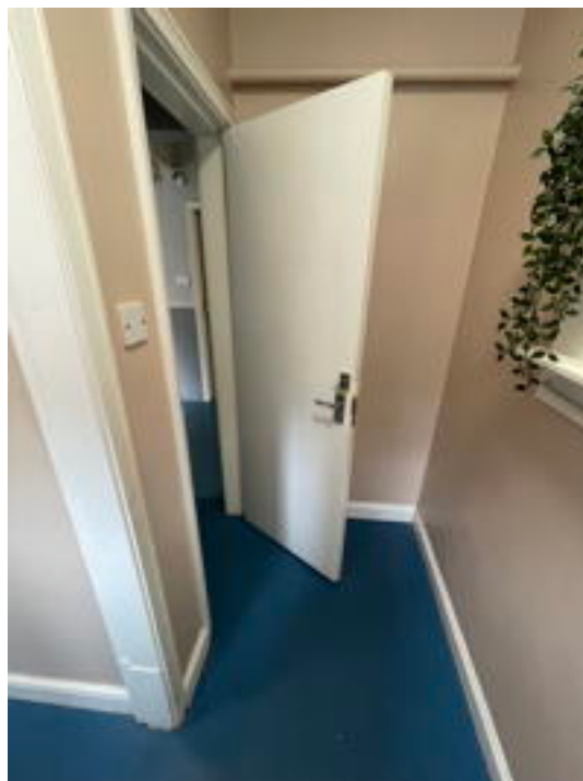
WC Looking North
