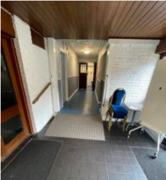
Hall Link Lobby Looking East
