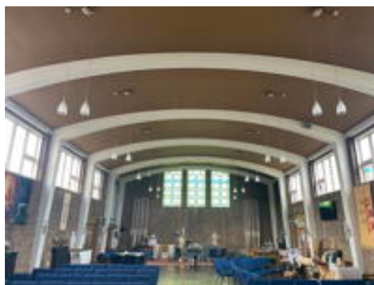
Roof Looking West
