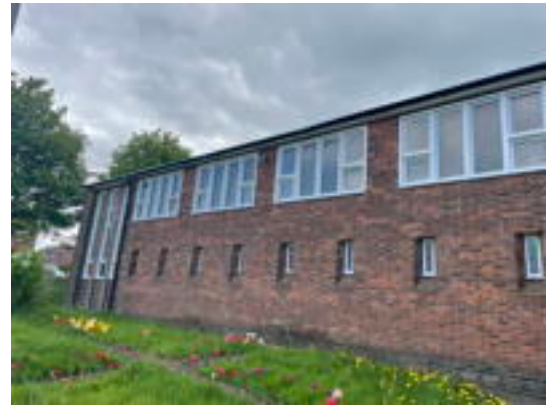
North Elevation Windows
