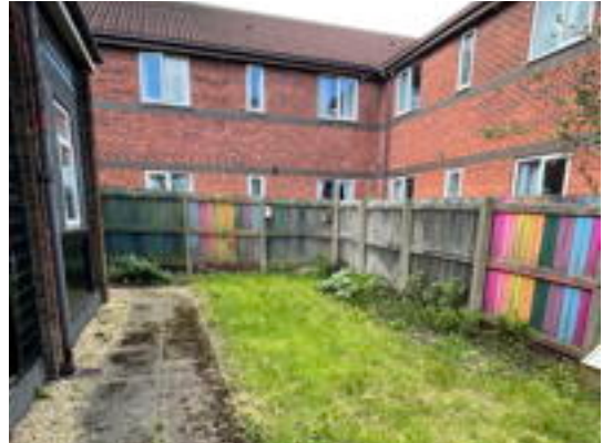
Fencing South West Corner
