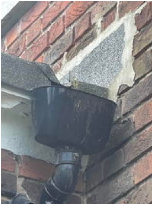
North Porch Lobby Hopper Head
