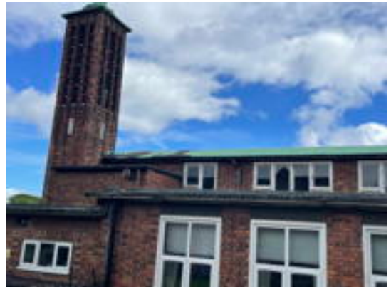
Patching to South Elevation Roof
