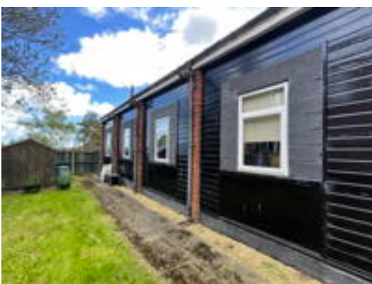
Hall West Elevation Windows
