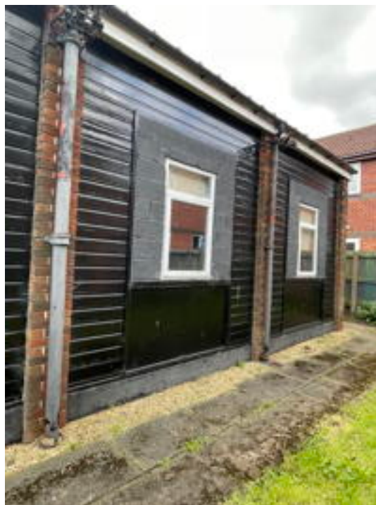
Hall Rainwater Pipes
