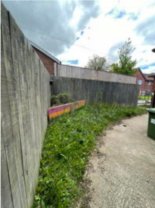
Fencing South East Corner
