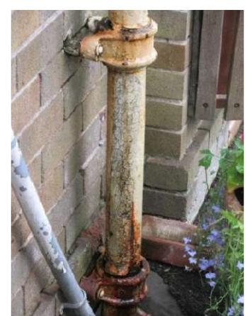
36. Two high Tower outlets have hoppers and long pipes, sound but very rusty especially at pipe backs, although held well off walls so not hard to paint. One looks blocked.
