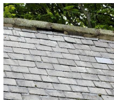
Figure 2 - South Chancel Ridge
