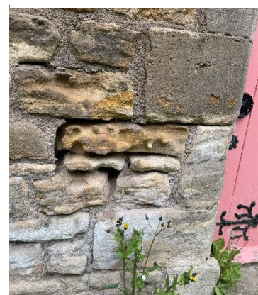
Figure 13 – South Tower First stage
