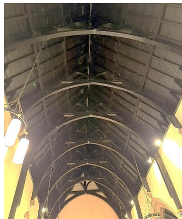
Figure 23 – nave trusses and boards
