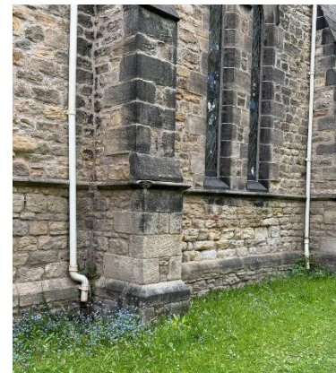
Figure 8 – South Nave RWP short
