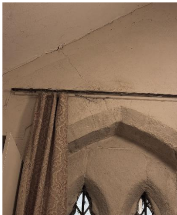
Figure 27 - Vestry crack
