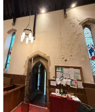
Figure 28 - West wall, near door
