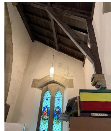
Figure 29 - N aisle, West wall
