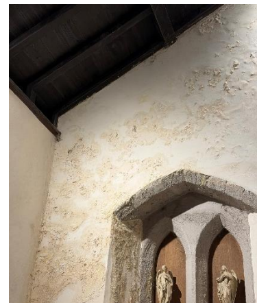
Figure 30 - Lady Chapel, east wall
