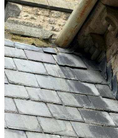
Figure 4 - Porch East ridge
