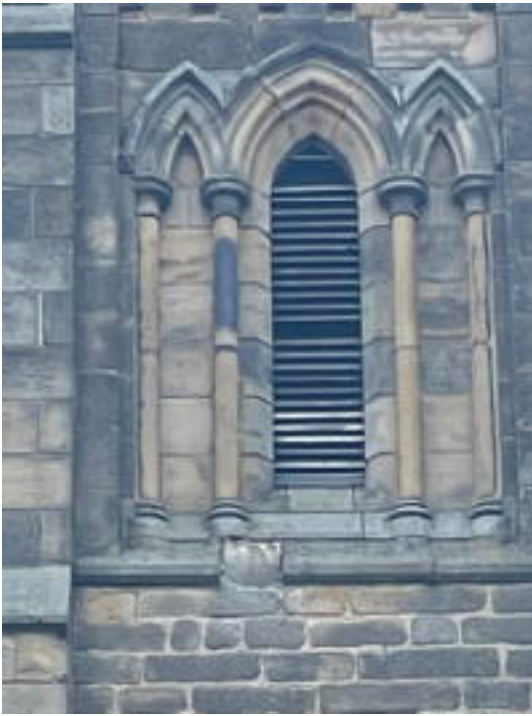
Tower Fourth Stage West Arcaded Triple Lancets, outer arches blind
