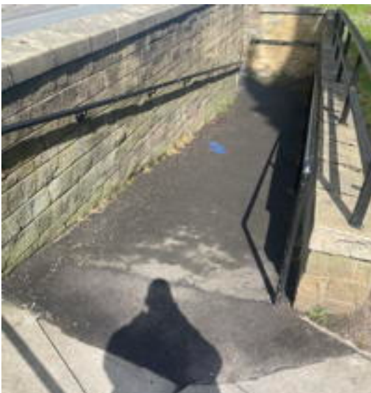
West Access Ramp
