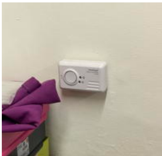
Carbon Monoxide Alarm
