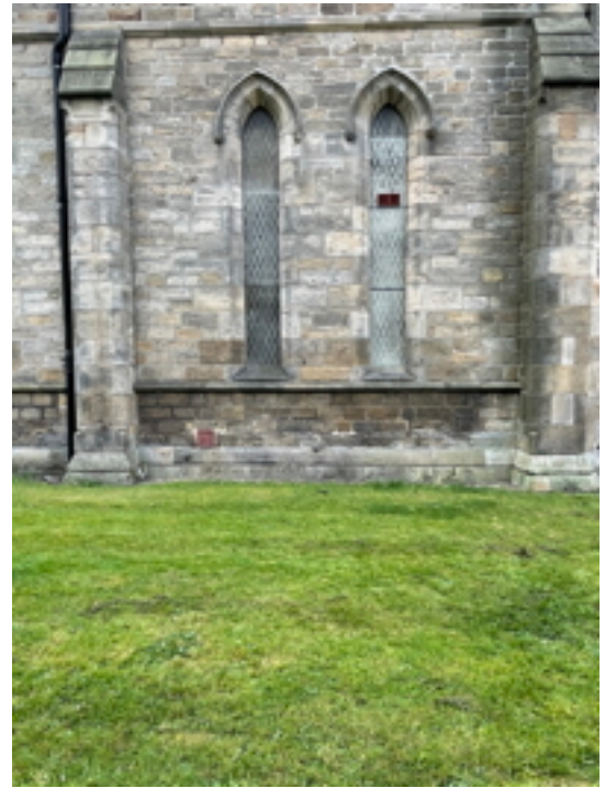
W3 and 4 Gallery Staircase Vandalite Security Glazing
