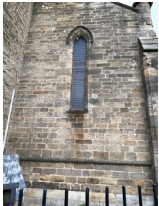
W27 Gallery Welcome Room West Elevation Obscure Polycarbonate Sheet
