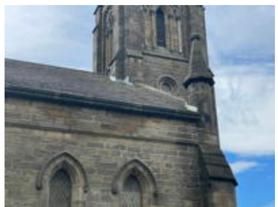
North Elevation West End
