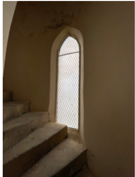
W1 Tower Staircase Vandalite Security Glazing
