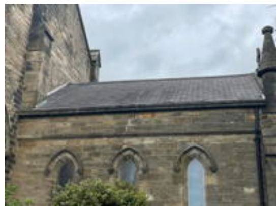
Chancel South Roof
