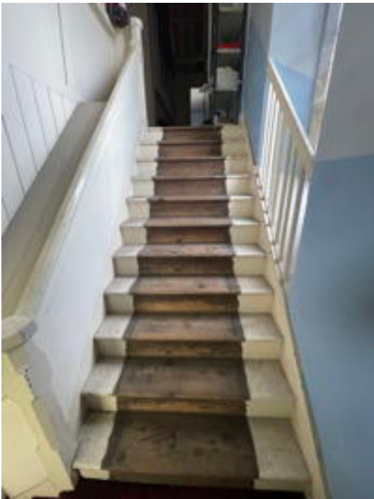
Gallery Staircase Looking South
