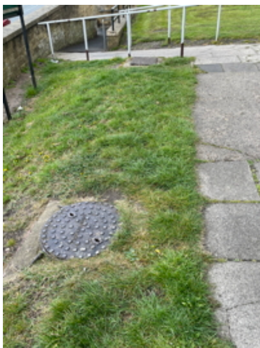
West End Inspection Chambers
