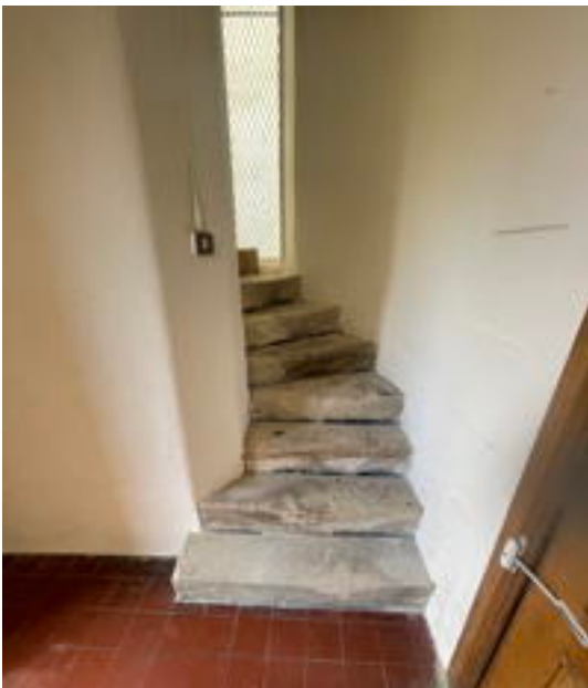
Spiral Staircase to Ringing Chamber
