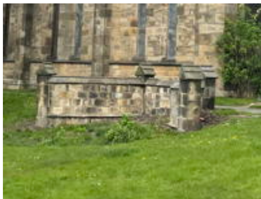
Former Boiler House Entrance
