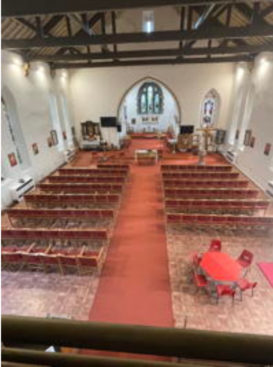
Nave Floor Looking East
