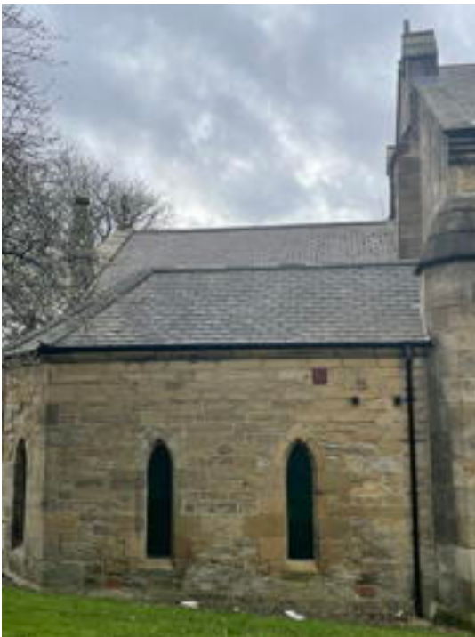
Vestry and Chancel North Roof
