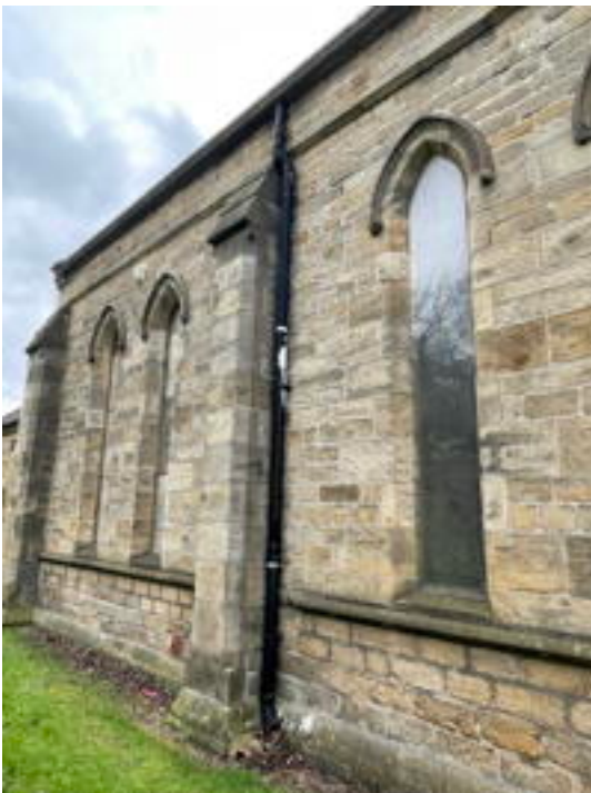
North Elevation RWP
