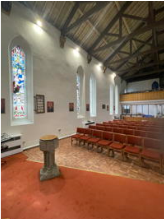
South Elevation Wall
