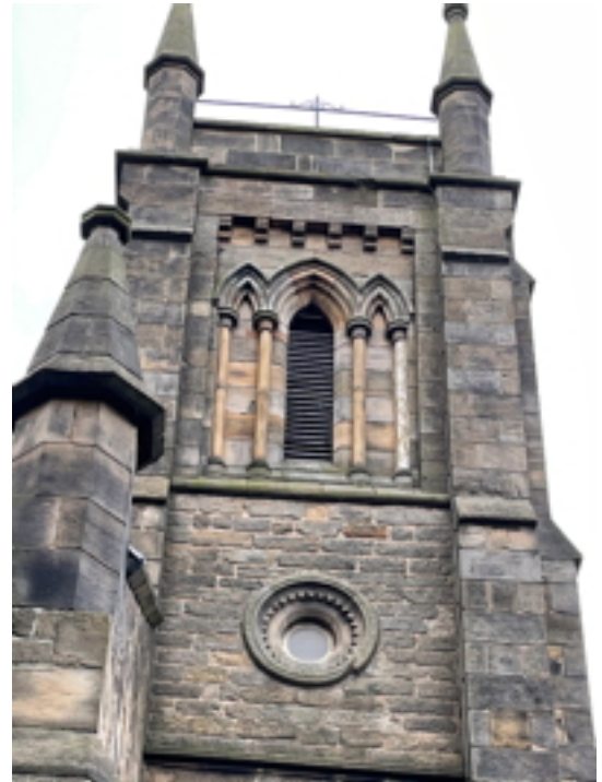
Tower Fourth Stage North Arcaded Triple Lancets, outer arches blind
