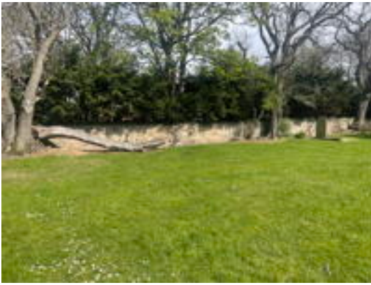
Grassed Area to the North
