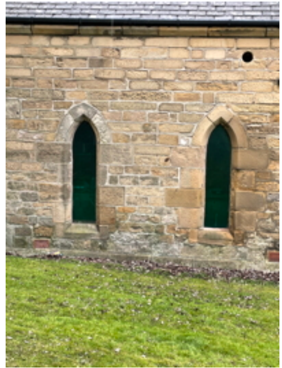
W11 and 12 Vestry North Green Film over Polycarbonate
