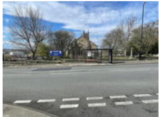
East Elevation Wall Missing Pointing, Plant Growth and Rusting Railings
