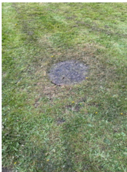
West End Inspection Chamber
