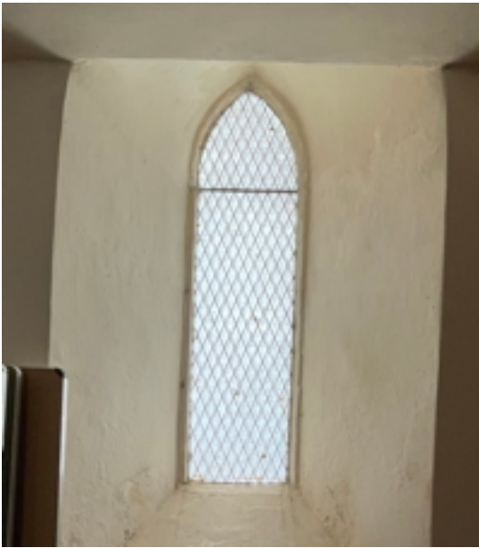
W28 Porch South Window Vandalite Security Glazing
