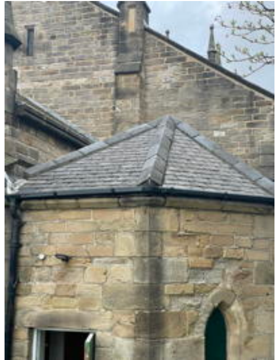
Vestry East Roof
