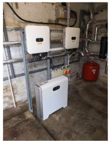
The PV panels have been installed comprising thirty 370W panels producing an 11.1kWp PV array generating 10,383kWh per year. This has been sized to best correspond to the schools electrical usage and is expected to have 95.3% of the energy generated used on site by the school thus avoiding export. To achieve this the system has been installed with a 5kW battery. The invertor and battery system were supplied by Huawei and are the first installation of this kind in the UK.
