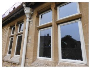
and very high draught levels within these rooms (as the previous top opening lights failed to close properly), the new windows are also much easier and safer to open and allow increased levels of ventilation into the rooms when open, which help to address summer time over heating and high ventilation levels to reduce viral risk.
