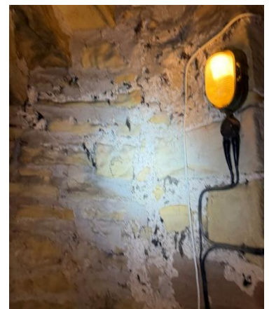
Figure 42 - Plaster to stair
