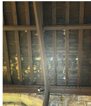
Figure 53 - E end S Aisle
