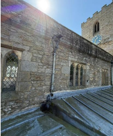
Figure 19 – N Aisle w/ Nave outlet
