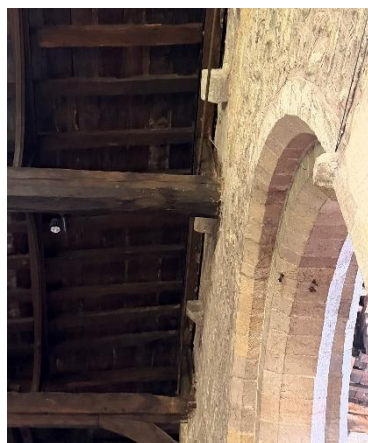
Figure 51 - N Aisle wallplate S
