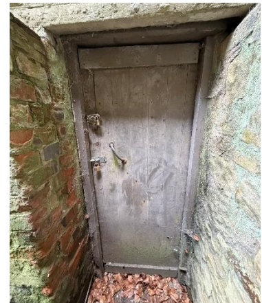
Figure 45 - Boiler room door
