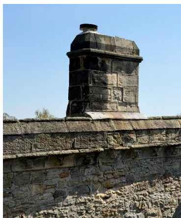
Figure 29 - W Vesty chimney
