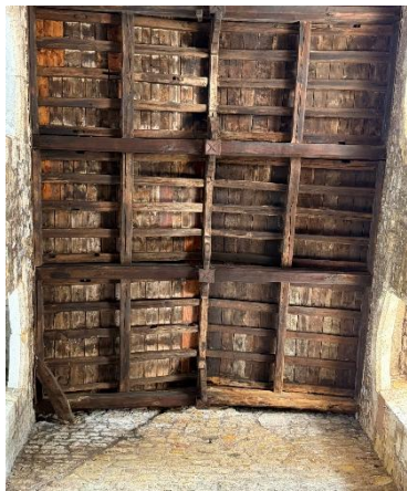
Figure 49 - Nave roof overall
