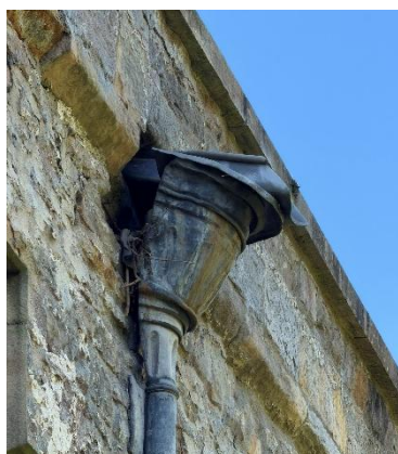
Figure 22 – N Aisle hopper
