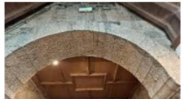
Stable and cracking is the same as the last QI: West 3mm, N 2mm at keystone. Slight amount of pointing fallen out of the southern arch but no action required.
