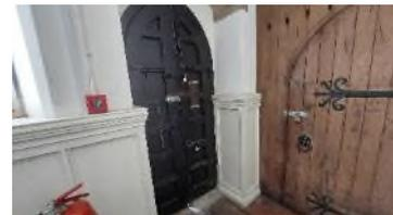
Some water penetration in the past on the choir vestry side, perhaps is condensation? Wind blowing detritus through the doorway, the door itself doesn't close adequately even though it is adequately bolted up but it does let in rather a draught.
