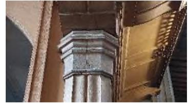
This contains the yurt and it rather fills the space but it is a successful addition to the Minster. Trip at the doorway. Shrinkage to W capital gallery column. Separate electric heater. This is a possible fire risk in a flammable structure that could imperil the building. The same thoughts go with candles if they are used and so a management system needs to be in place to reduce risk.
