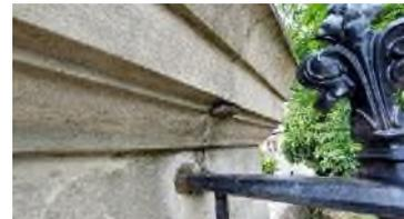
The twin gates have been redecorated but have no ironmongery or restraint. The sandstone pier caps have been replaced. There is rusting metal still in the piers which should have been removed. This entrance no longer makes sense- it was for when the church was accessed at the west end and so to use it makes for a dog leg path within and an indirect approach from The Green.
