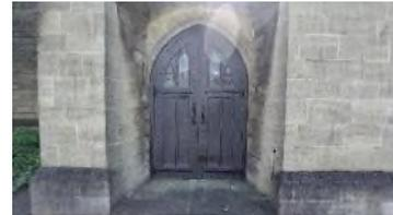
North Side – Open joints at higher level to the parapet and the eastern buttress, slight chipping to two of the coping stones. Generally the wall is ok. Two light square head window with rusting ferramenta with dirty polycarbonate. Pair of heavy double doors. Decoration fading now, rusting to the hinge pins and to the hinge braces.
