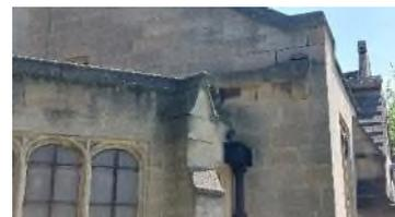
Open joints to the parapet top and the buttress on the north west elevation. Three sets of windows with rusting ferramenta and polycarbonate that is dirty.
