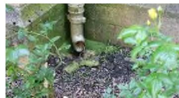
Three downpipes with ornamental hopper heads (hoppers repainted in 2018) and anti-climb paint is wearing away a bit at the upper levels. The remainder of the pipes coming down to the ground look sound, Middle pipe blocked at inspection ( and cleared) .These all discharge to gulley's that should be checked to be clear of blockages
