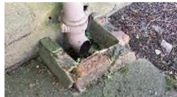
South Side – A mixture of old and new half round gutters. The decoration is coming away as is the joint between them. Rusted out at the back. Anti-climb paint on the upper part of the downpipe appears ok. The bottom part of the downpipe's decoration is coming away and it's a little bit high for the gulley but it will do, the gulley has leaves in it.
