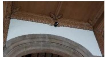
No real change here from the last QI report. The flat ceiling is unblemished. The walls have some lead sulphate marking particularly to the south side at the lintels. The walls are in good condition and there is no cracking to the arches that look onto the chancel and to the south inner aisle. Flooring is a mixture of herringbone and floor slabs.
