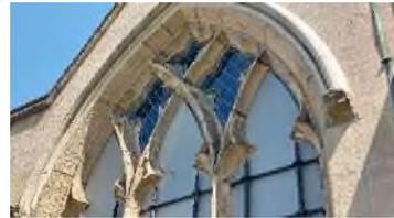
Generally the walling is sound, and interestingly, this is the only part of the 1930's work where Caroe has retained the original sandstone (apart from the tower) at the bottom of the central window and this is shaleing slightly.
