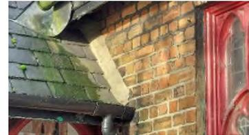
Same style as the nave, except the ridge tiles are grey. Slating both sides are ok. The mortar abutment flashings are sand cement covering the lead work to discourage thieves.
