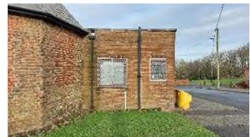
**South side –** Same erosion. The window head is soldier courses unlike the flat arches elsewhere, open joint at the angle change.
