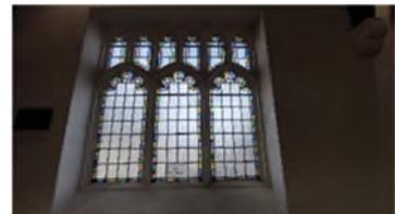
Most of the glass is obscure leaded with coloured margins, it does look a bit dirty on the polycarbonate, quite a lot of condensation on the glass. One pictorial window on the south side to the Bradley family, the condition is good.
