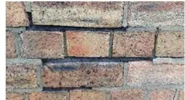
This is a small part that is left over from being enclosed by the hall, brickwork a bit patched, cement pointed, some open joints, some bricks losing their face but in fair condition.
