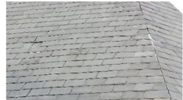
**North side** – Octagonal hipped ends with cut mitres. The abutment to the nave gable has some loose and cracked slating. Probably caused when accessing the roof to steel flashings. The chancel abutment flashing to the nave gable looks to be just mortar, I don't know that there is any lead behind it.
