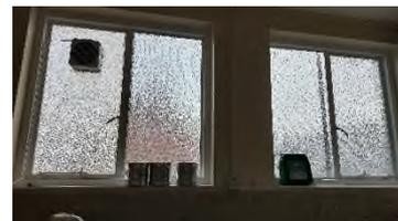
Catering standard. Ceiling and wall decoration is ok, floor is good, contains good appliances, there are windows on the east made of obscure glazing they are not easy to open as they are rather high and is painted up now, condensation on the glass, high level borrowed light windows look ok. Is extract fan adequate?
