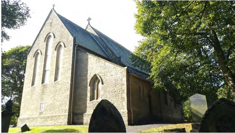
Welsh slate looks ok as do the lead flashings up the head and the abutments. Watertable to E end looks ok. Organ loft Westmoreland slating with tingles some replacements I think it is all sound. Ridge flashing in new lead against the nave looks good. W abutment mortar over lead ok. E abutment rather heavy handed looking mortar pointing over probably lead. Looks like there is some silicon type pointing to the watertable.
