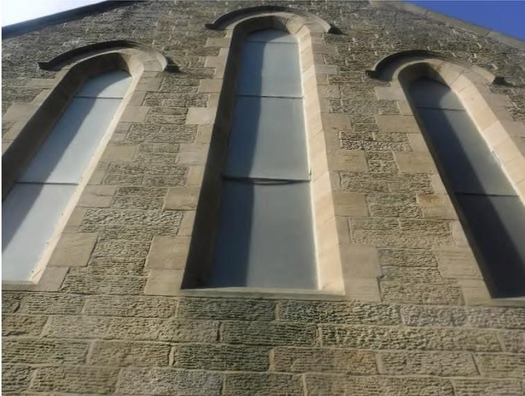
**South side** – Two single lancets has seen movement at the western arch top but ok, within are unprotected clear glazed lead quarries with rusted ventilators.
