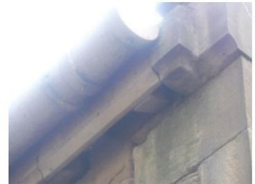
**Recommendation:** replace plastic with cast iron, redecorate. Unblock gullies, repair broken fittings, adjust outlets to drain into gullies, clear blocked downpipes, improve leaf guarding at gullies
