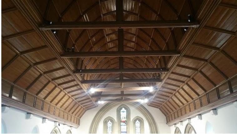
The nave has a wagon style roof faceted boarded ceiling with ribs at upper and lower level, The decoration colour and gloss finish doesn't contribute to the recent reorder.
