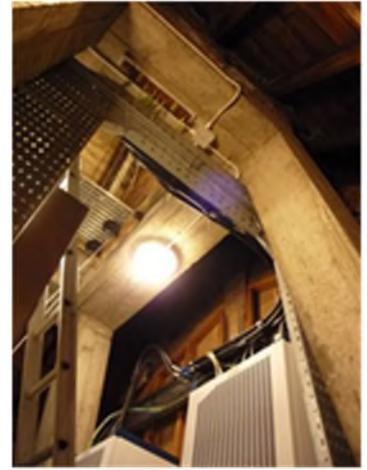
**C** The general installation of the electrical cabinets, which appear to be for both Vodafone and BT, appears okay. The incoming service cable infill is poor and letting in a draught.
