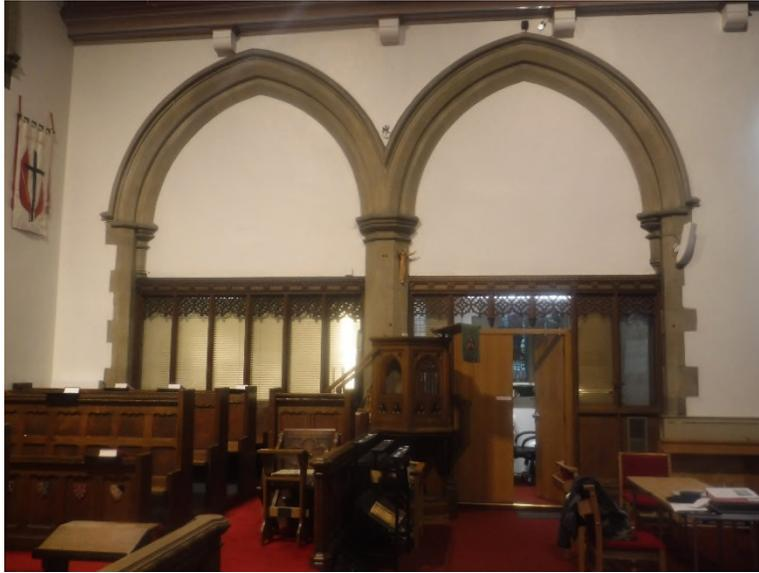
Slight fracture to the arch stone closest to the E but hairline is just an easing, the other arch is ok, and down to the ground the arches look sound.
