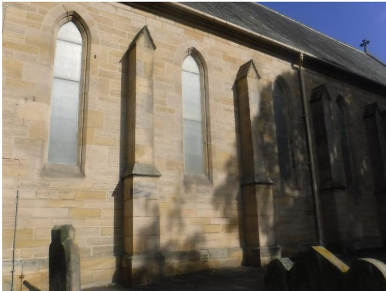
**South side** – Eaves cornice ok, walling is sound repointed rather heavy strap pointing but it is ok. Buttresses have little apex roofs and whilst they have got some minor open joints they are ok.
