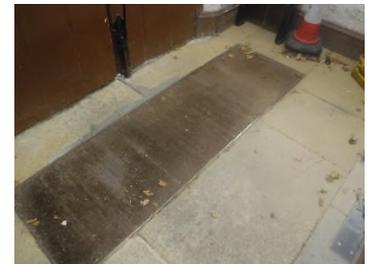
**Porch vestibule** – Some open joints in the paving slight trip hazard of the galvanised edge to the mat well itself which is worn out now and could do with being renewed.
