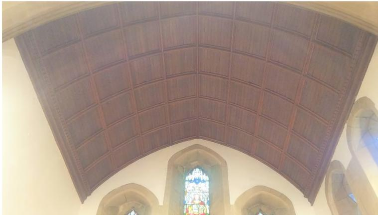
The chancel has curved lancet style roof with ribs and timber boarding, no water marking, it looks like the original finish and it is very good compared with the nave
