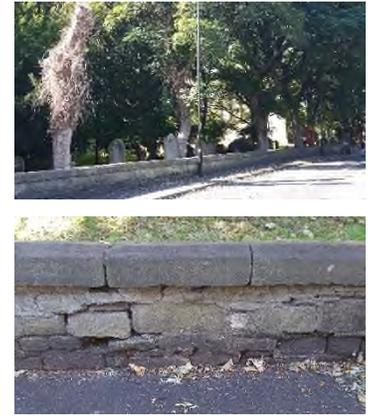
Low wall retaining the sloping churchyard and there are many open joints to it at low level. To the NE end is a pillared entrance without gates. Paths are tarmac and ok.
