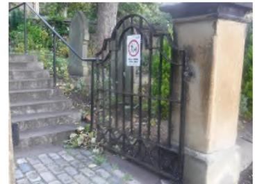
Steps continue to be buckled a little at the lower stage and there are open joints. The gates don't open as they are rusted up. To the N side of this the low wall is cracking in a couple of places.
