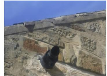
Welsh slate covering that is all ok, has had new lead ridge flashing up against the nave. West abutment to watertable ok in mortar. Poor overhang verge at the E end and there is some breakdown of the pointed verge. It'll probably last a while so save it up and then remake the verge properly in about 10 years.
