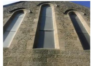
**South side** – Upper part matches the nave but the majority of the wall is in random rubble and badly smeared with pointing and a couple of eroded stones at the bottom but generally sound. Cotoneaster up against this so can't see behind that very well, there is some erosion I think.
