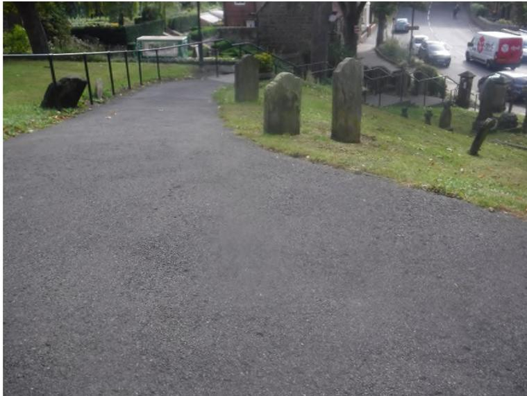
Comprises burial ground, multiple headstones and mature trees. Steep path to the W, S and E. They are tarmacked and have hand railing which is sound. The entrance area has paving and handrails with open joints to the stonework which was due to ground movement from the installation works and now is being caused by tree root movement.
