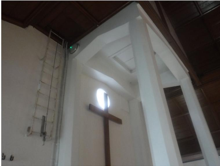
The belfry is supported by a concrete structure which is made up of octagonal columns which go from the roof down to the ground, they look ok, there is no cracking to the support to the gallery either.
