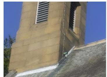
The N W corner is doing the same, (not reported in last QI- was it missed?). Minor erosion to the pointing as before. Spire copper looks ok and the bent E symbol of the weathervane remains bent. It is quite windy today and the weathervane itself isn't rotating. When the lightning conductor people visit they should have a look in the base of the spire and also the roof arrangement of the belfry.
