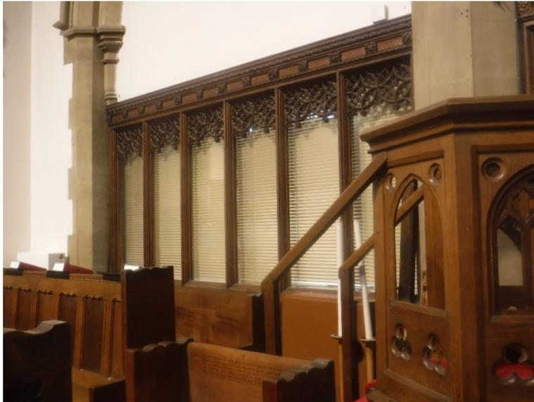
Oak partition screen with fine fret work, fine fret work, good cornice, retro glazed in good condition, it has had a rather poor looking door inserted into it, it is just a flush door and rather beaten up. The inside of the panelling is less decorated but ok.
