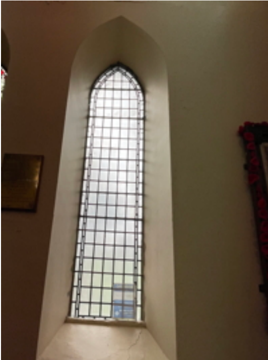
Window 1 Leaded, plain glass, good condition
