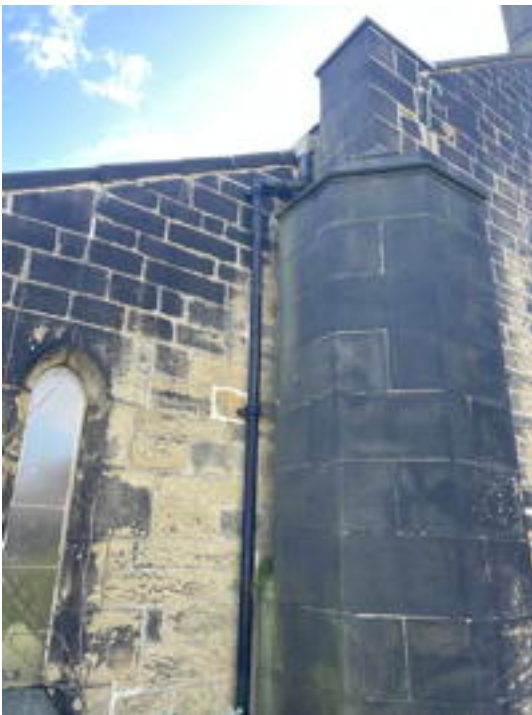
North Aisle West Rainwater Pipe
