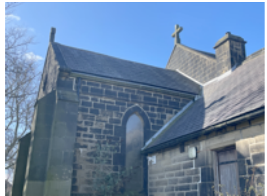
Chancel North Roof
