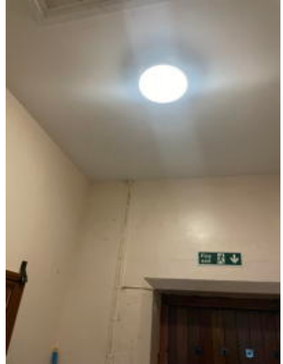
East End Lobby Looking East
