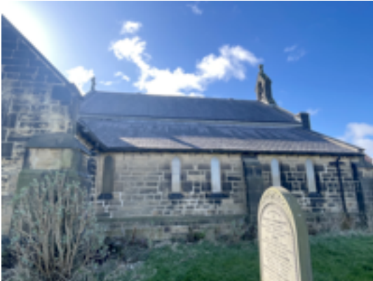
North Aisle and Nave Roofs
