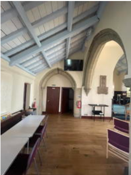
North Aisle Oak Flooring
