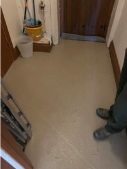
East End Lobby Looking East
