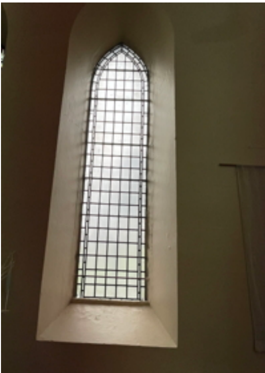
Window 3 Leaded, plain glass, good condition
