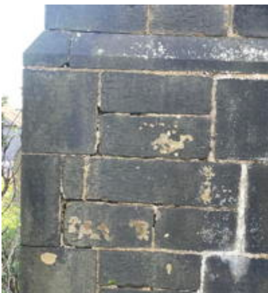
Vestry West Elevation Pointing
