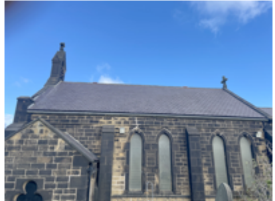
South Nave Roof
