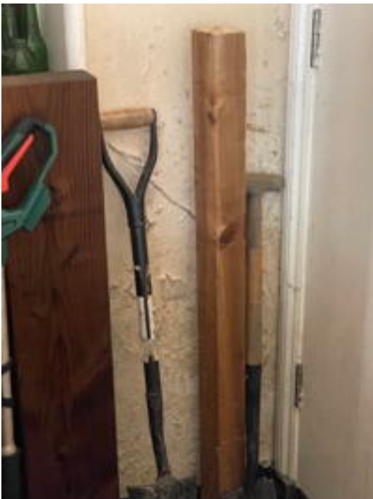
Deteriorating Paintwork South Wall
