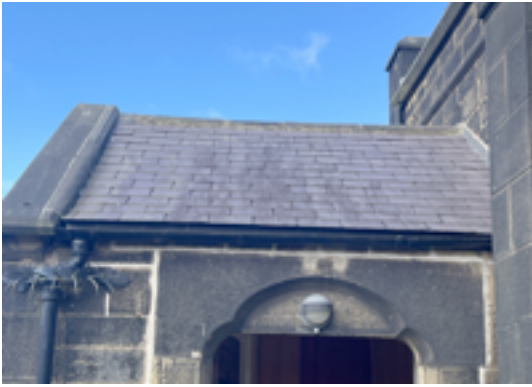
Porch East Roof
