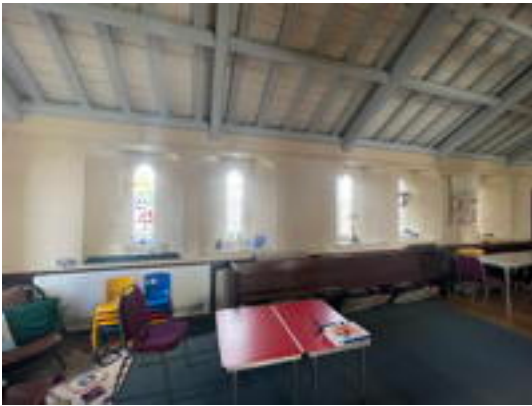
North Aisle Pews
