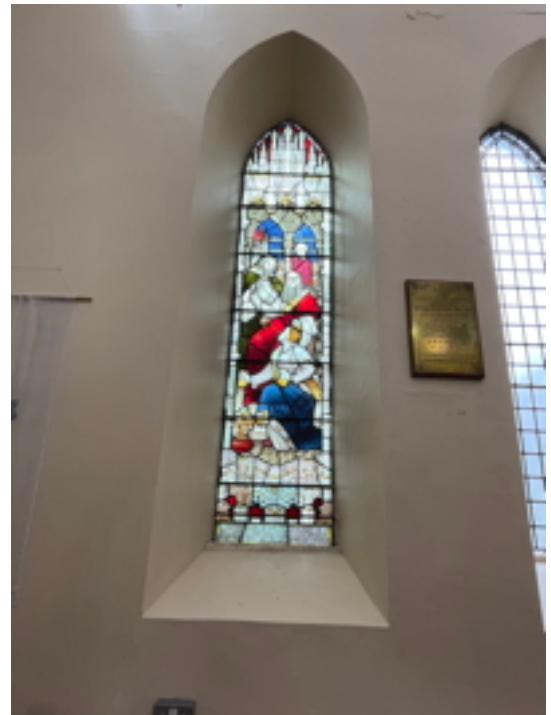
Window 2 Stained glass dated 1901, satisfactory condition
