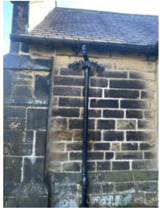
Vestry West Rainwater Pipe
