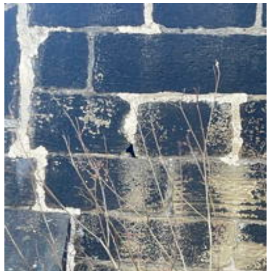
North Aisle West End Pointing
