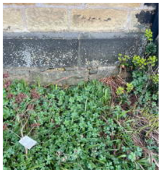
Chancel South Elevation Pointing
