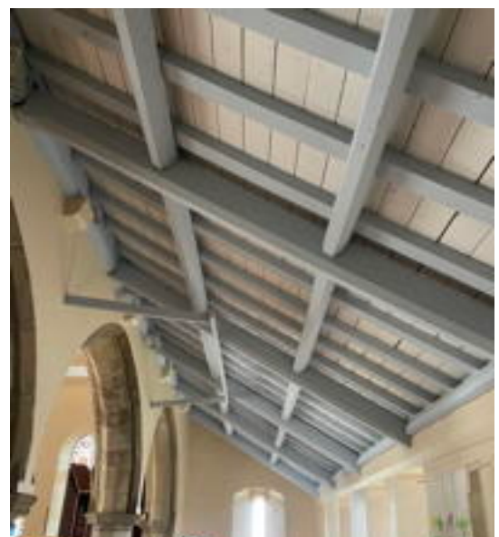
North Aisle Roof
