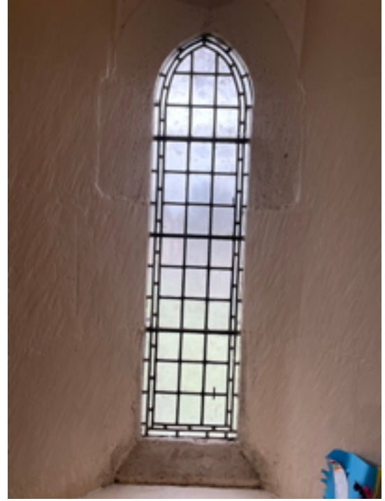
Window 18 North Aisle, single lancet, plain.
